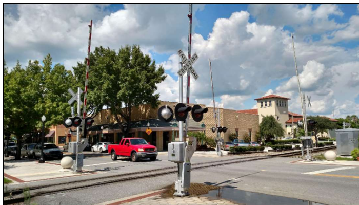
Railroad crossing in Lakeland, FL.
