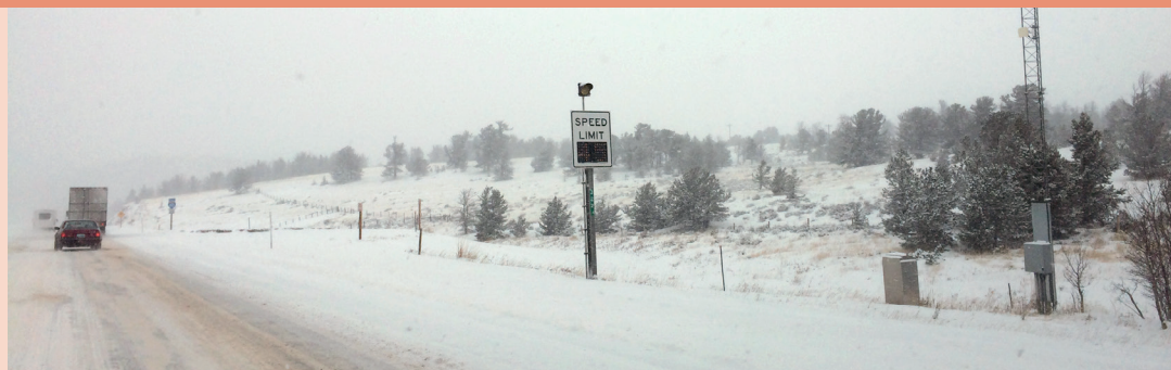
I-80 – Wyoming Variable Speed System, December 2014 Photo courtesy of Dr. Mohamed M. Ahmed, PE, University of Wyoming
