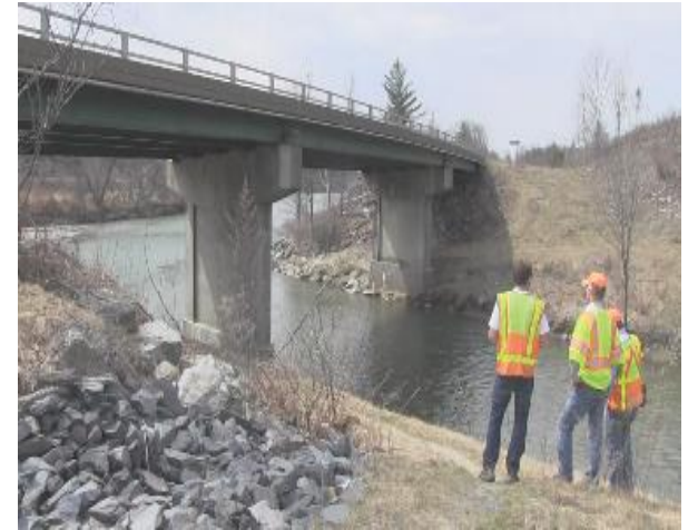
VTrans Bridge Program staff at a project site. (VTrans)
