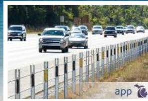
MDOT Guardrail App
