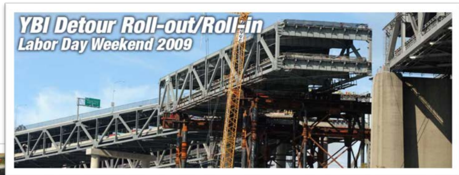
SFOBB Yerba Buena Island Viaduct superstructure roll-in
