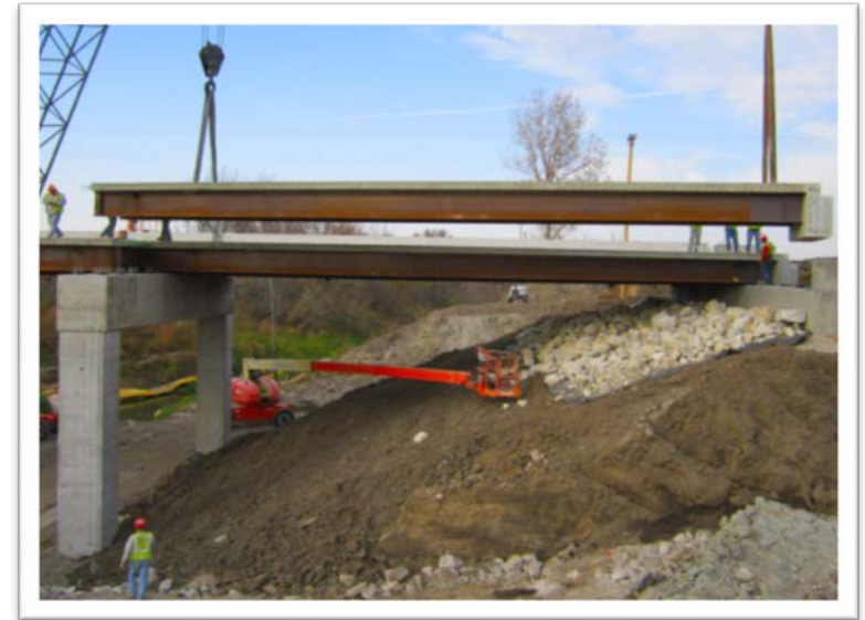
Bridge installation over Keg Creek, Iowa.
