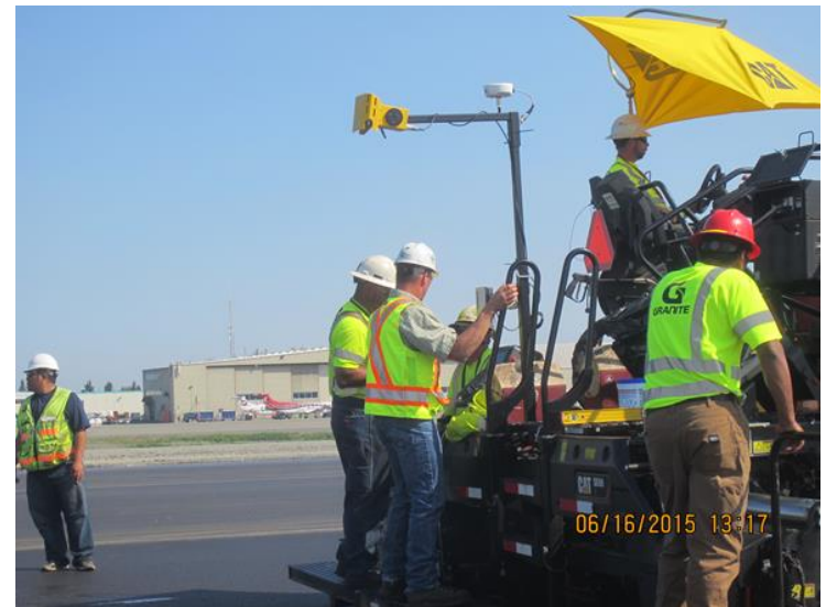
Testing at Anchorage Airport Project
