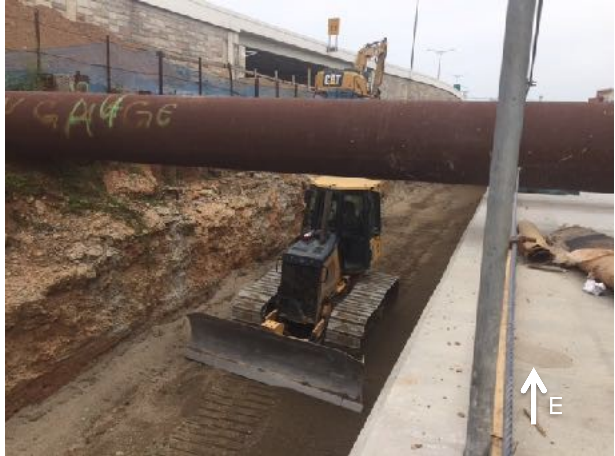
Backfilling to Final Grade
