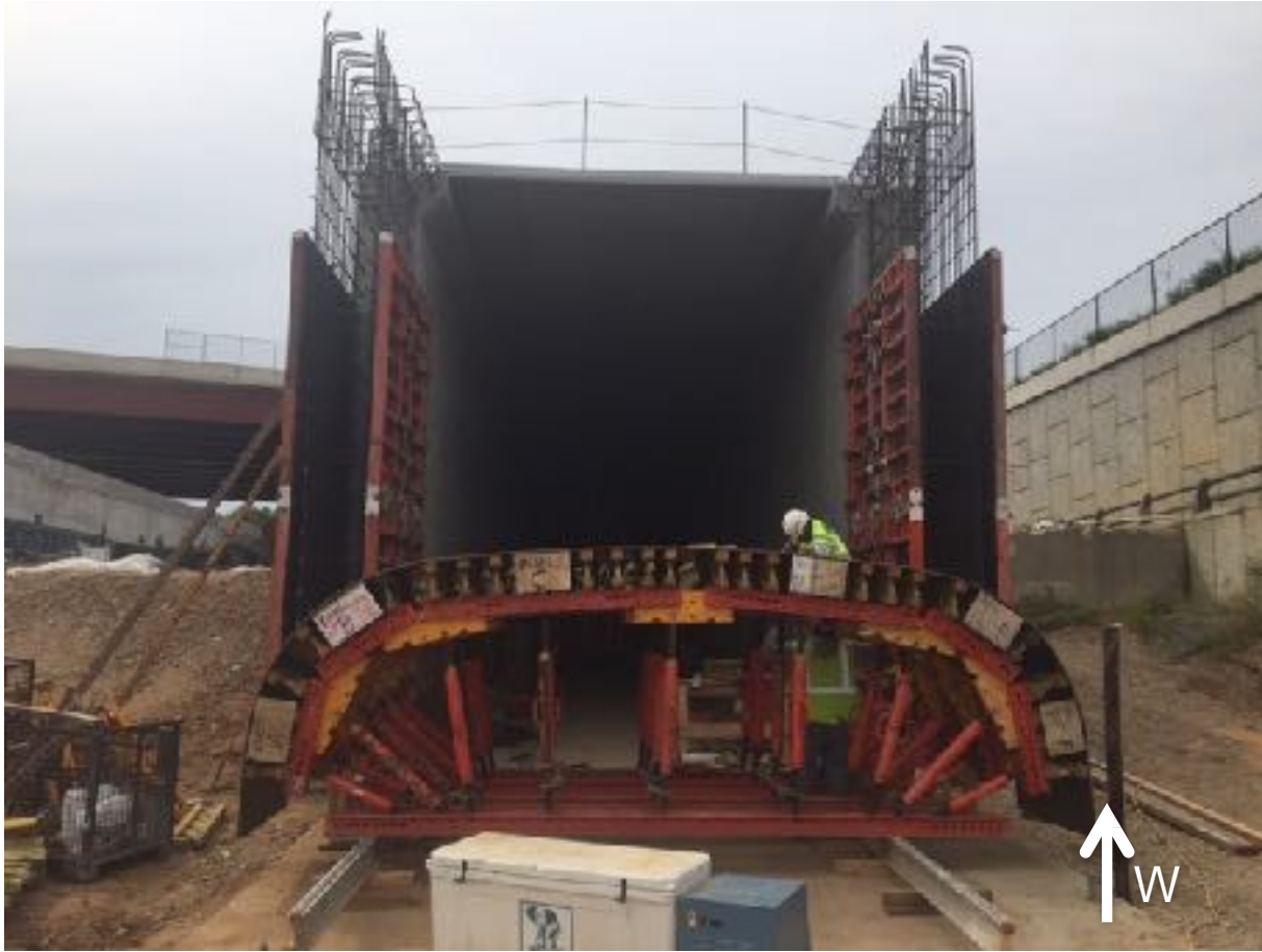
Forming Tunnel Portal
