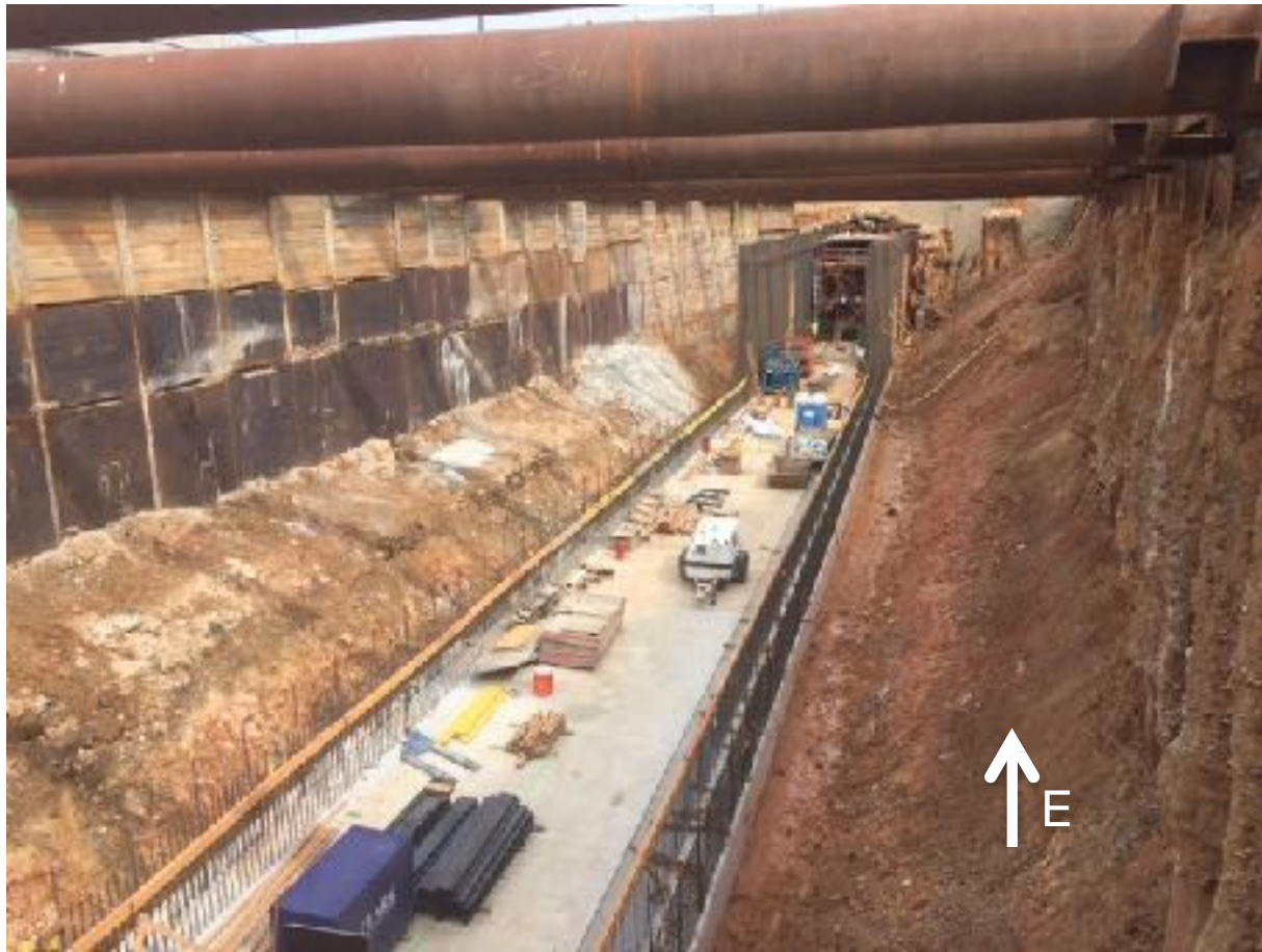
Tunnel Inverts and Walls
