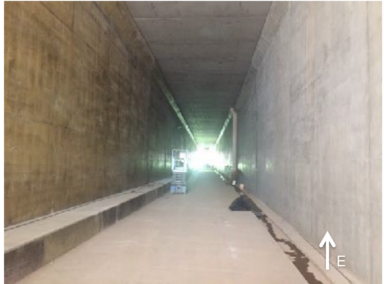
Inside the Tunnel
