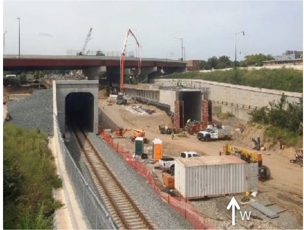
Pouring Concrete Roofs
