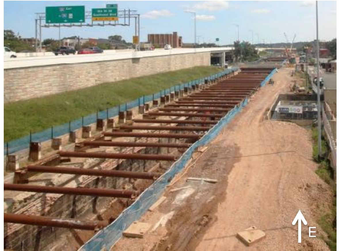
Tunnel Demolition and Excavation
