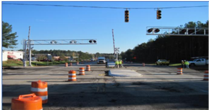
Construction of crossing signalization with traffic signal preemption installed under NCDOT's master agreement with Norfolk Southern Railway as part of a roadway widening project along NC 42 in Clayton, Johnston County, North Carolina.
