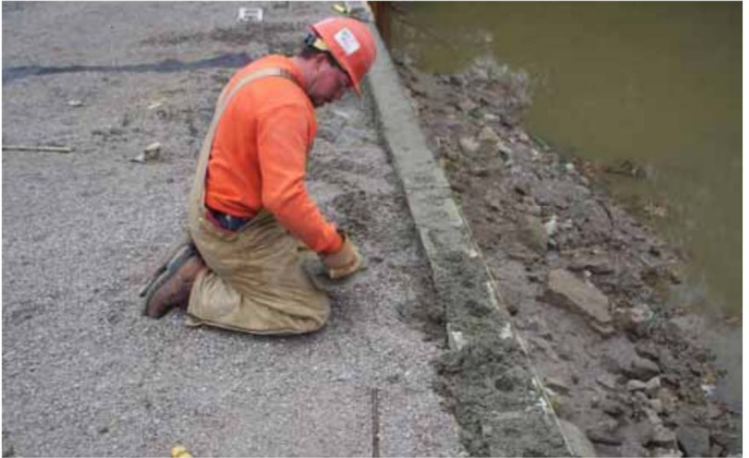
Figure 60. Photo. Connecting the top courses of blocks.
