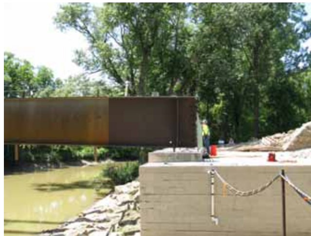
Figure 71. Photo. Steel girder on CIP footing.
