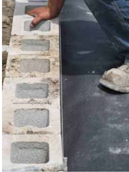
Figure 54. Photo. Checking block alignment with string line reference from back of block.
