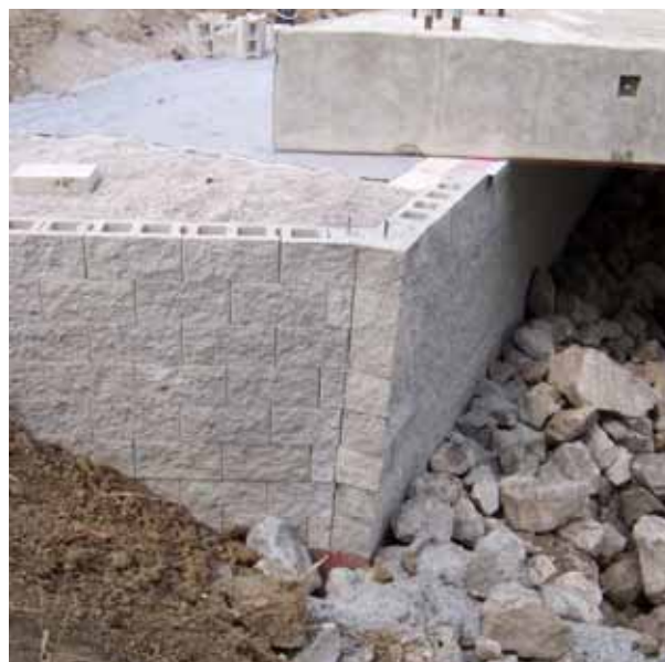
Figure 58. Photo. Vertical seam in wing wall.
