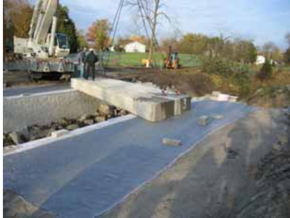
Figure 63. Photo. Box beam placed on beam seat.
