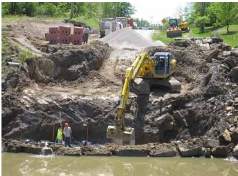
Figure 46. Photo. RSF excavation below stream level.
