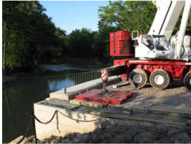
Figure 72. Photo. Outrigger pads near wall face.
