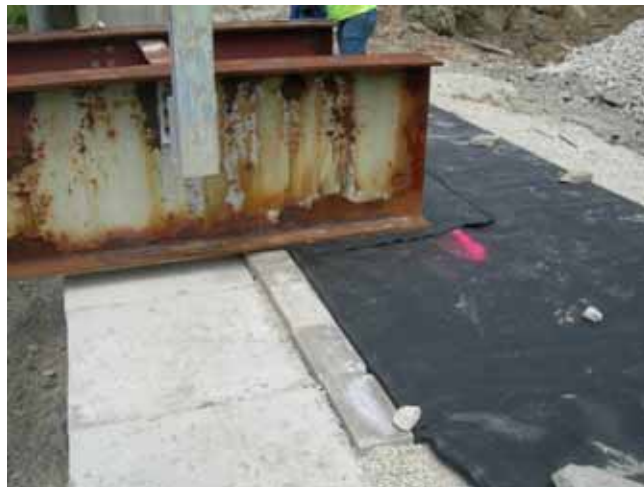
Figure 73. Photo. Additional reinforcement under beam.
