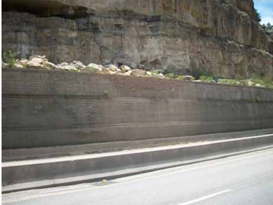
Figure 85. Photo. Repair of a GRS wall after damage caused by rock fall.
