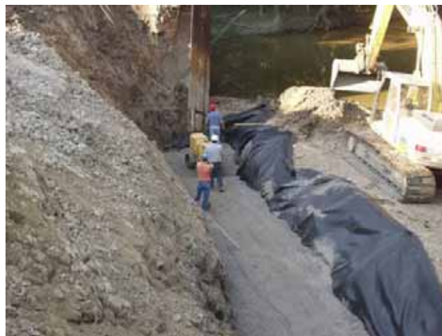
Figure 48. Photo. Encapsulation of fill in RSF.
