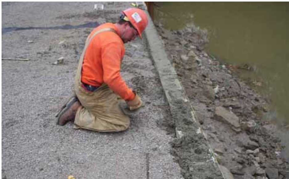
Figure 60. Photo. Connecting the top courses of blocks.
