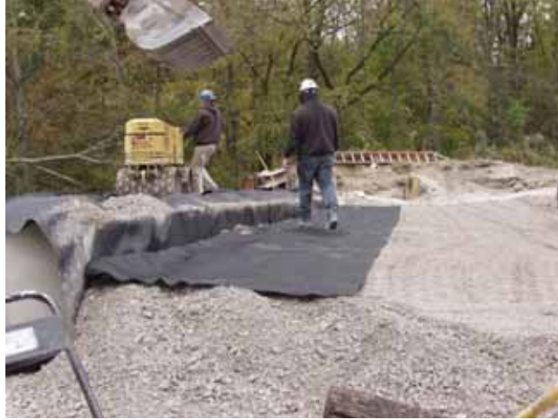
Figure 78. Photo. Secondary reinforcement sheet.
