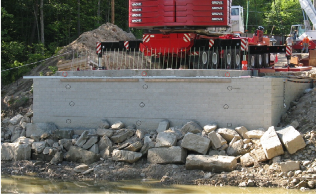
Figure 38. Photo. Location of survey targets on Tiffin River Bridge, Defiance County, OH.
