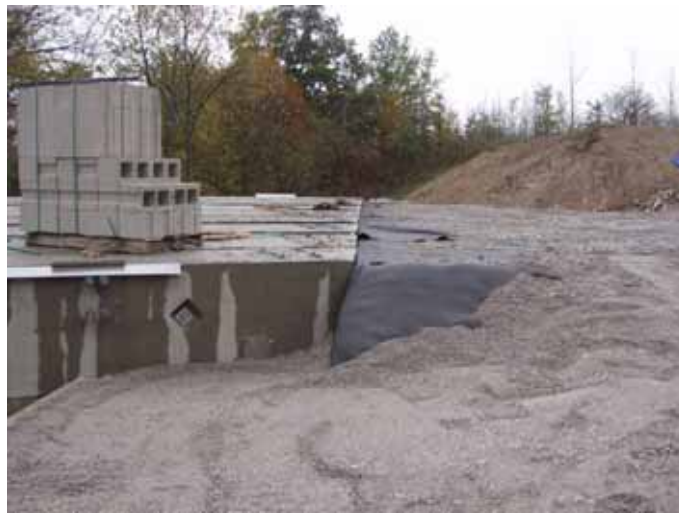
Figure 81. Photo. Completed approach fill.
