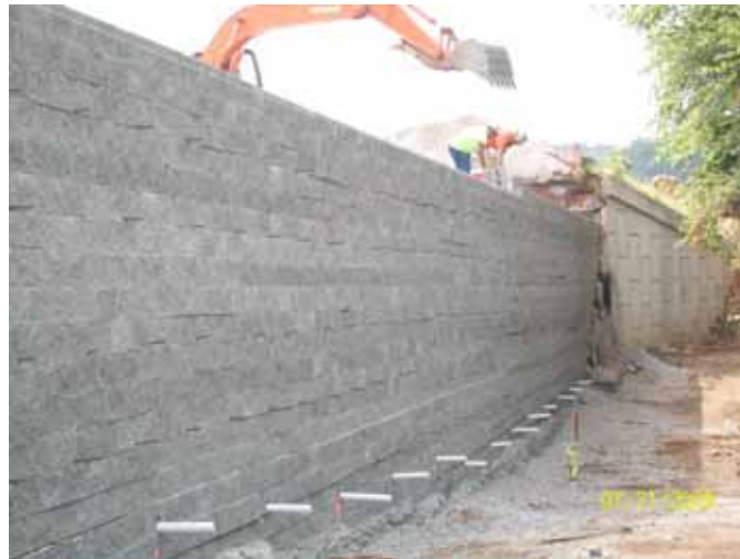
Figure 82. Photo. Use of GRS wall to repair damaged MSE wall.
