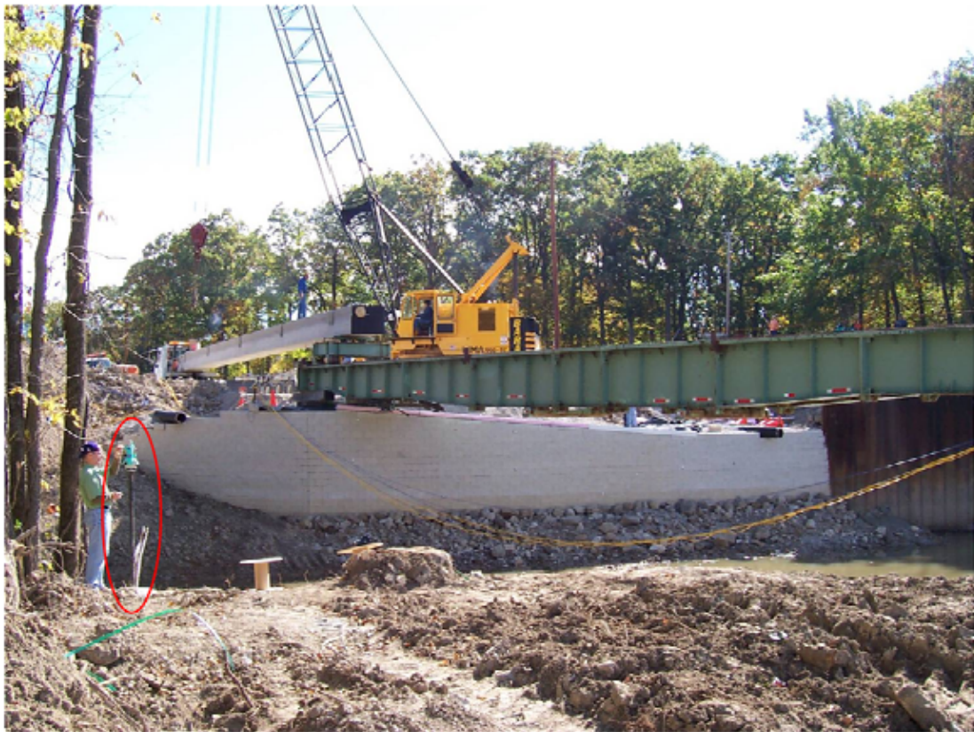
Figure 39. Photo. Location of total station reference pole.
