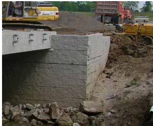
Figure 74. Photo. Parapet and wing wall construction, view 1.
