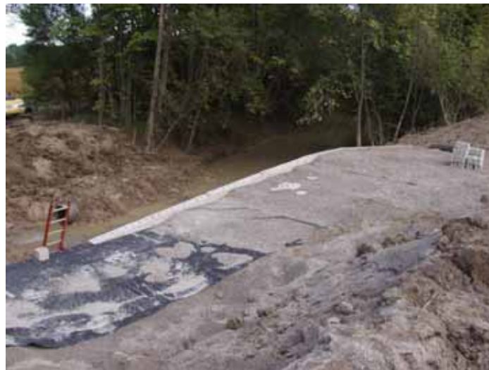
Figure 53. Photo. Superlevation reinforcement layers.
