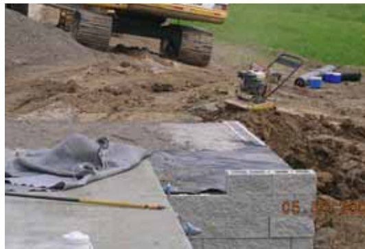
Figure 75. Photo. Parapet and wing wall construction, view 2.
