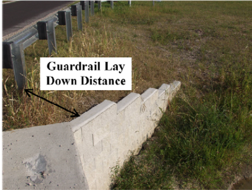
Figure 24. Photo. Guardrail lay-down distance.
