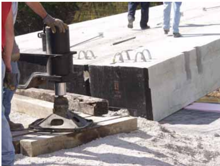
Figure 8. Photo. Bitumen coating on concrete beam ends.
