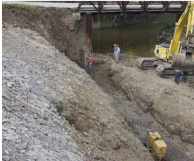
Figure 47. Photo. RSF cut preparation.
