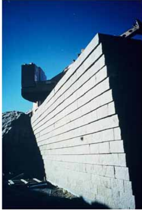
Figure 55. Photo. Negative batter wall face.
