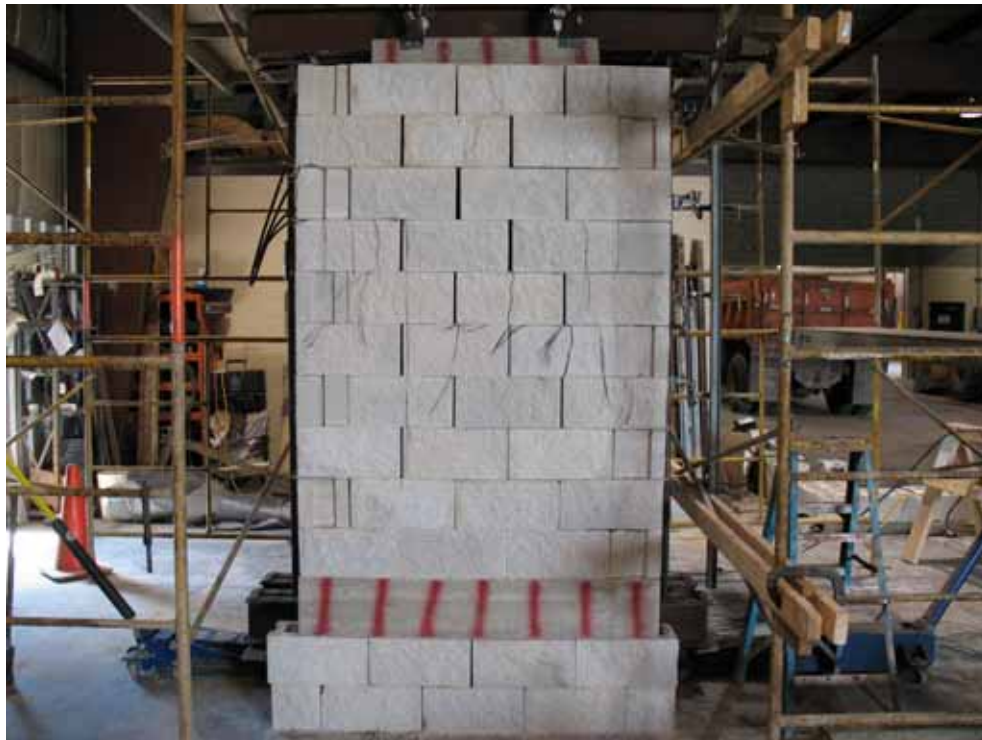
Figure 97. Photo. Defiance County experiment after testing.
