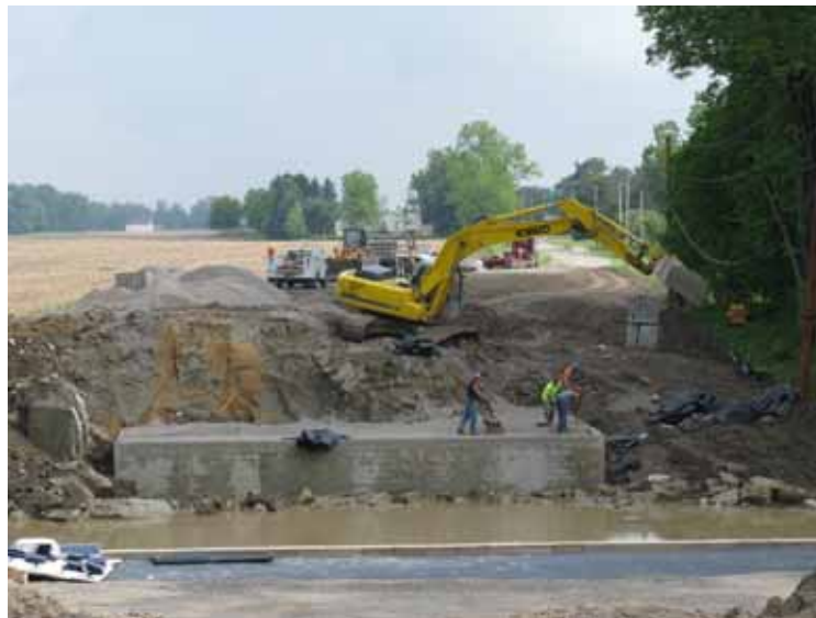
Figure 25. Photo. GRS abutment and wing walls built around core of native soil
