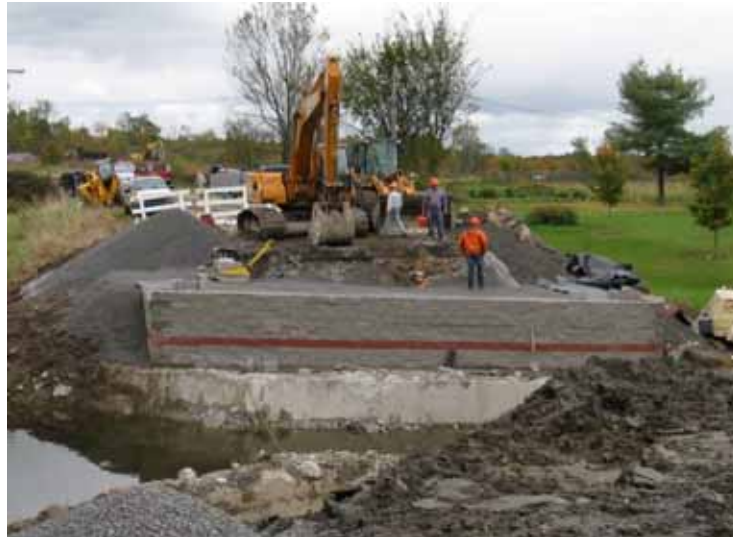
Figure 41. Photo. Cut slope of retained soil.
