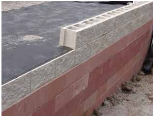
Figure 3. Photo. Split face CMU blocks.
