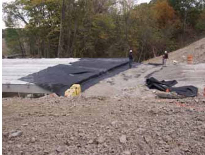
Figure 76. Photo. Placing reinforcement.
