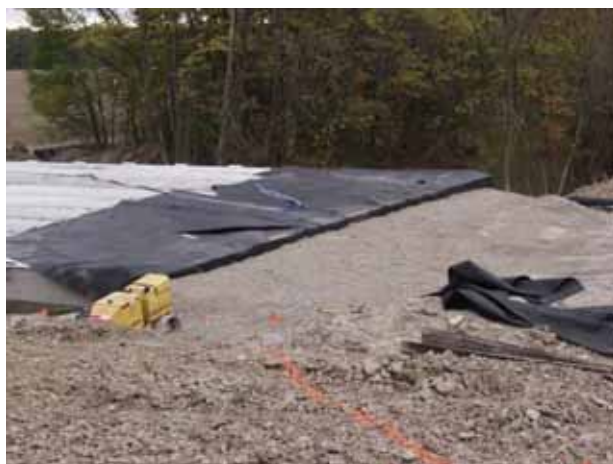
Figure 80. Photo. Second 6-inch fill lift.
