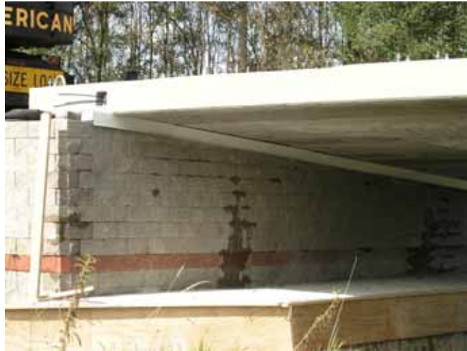
Figure 70. Photo. Aluminum flashing (drip edge) between beams and top of CMU block.
