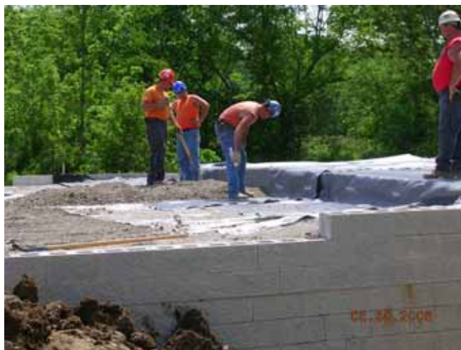
Figure 77. Photo. First 6-inch fill lift.
