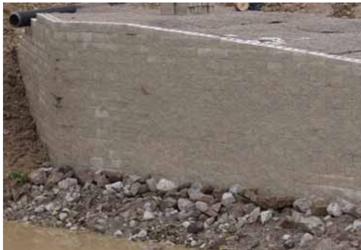
Figure 56. Photo. Blocks trimmed to match superelevation.
