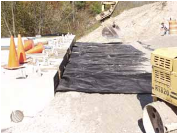
Figure 79. Photo. Completed wrapped approach layer.
