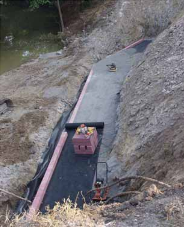
Figure 51. Reinforcement rolled out parallel to wall face.
