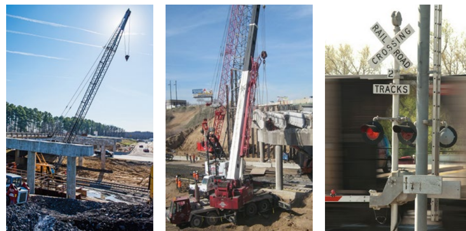
Photos Courtesy of: CH2M; Utah Department of Transportation.
