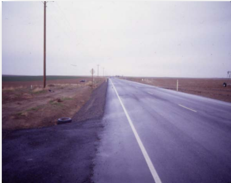
Example of segregated pavement
