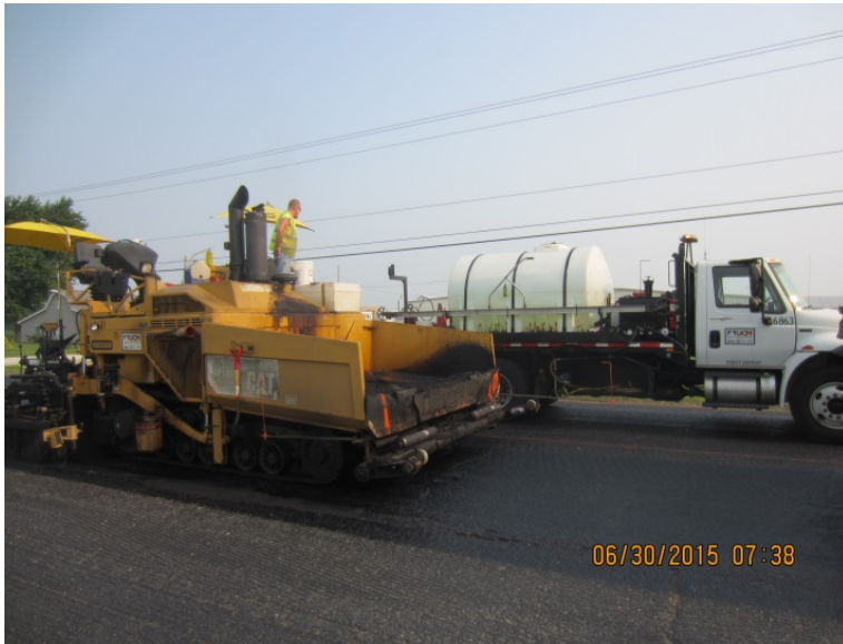
Mixtures placed with Caterpillar Rubber Tracked Paver
