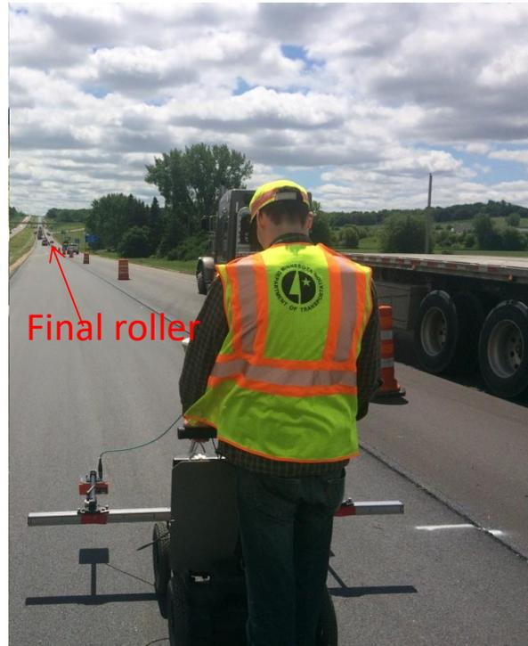
**Figure 6: RDM Surveying Behind Final Roller**
