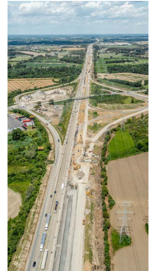
I-75 in southeast Michigan near Lake Erie | Photo courtesy MDOT
