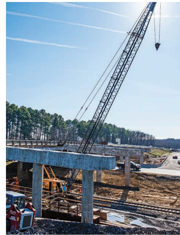
The Arkansas State Highway and Transportation Department is using tools from Railroad-DOT Mitigation Strategies to coordinate projects involving railroads. | Photo courtesy AHTD
