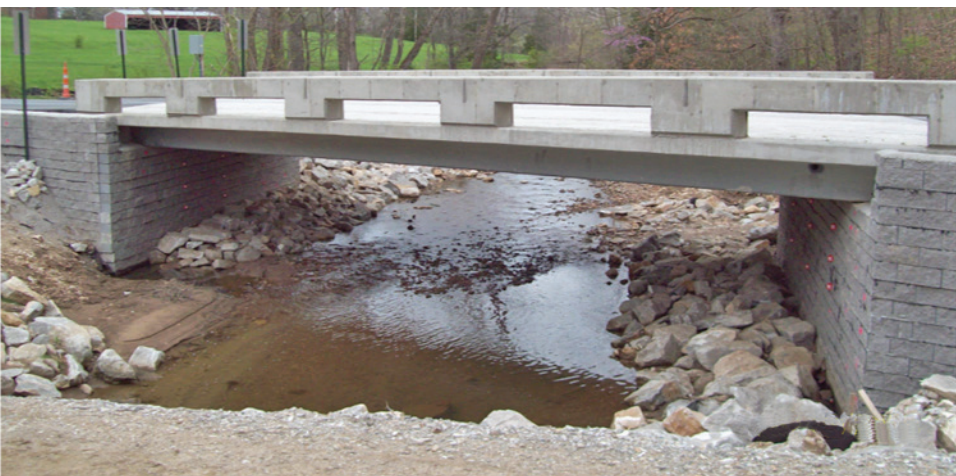
The completed Rustic Road Bridge, Boone County, MO | Photo courtesy Derin Campbell
