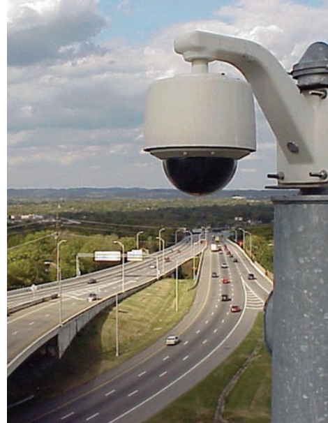
Since holding a TSM&O workshop in 2009, Tennessee DOT created a Traffic Operations Division, which uses cameras like this one to monitor traffic flow on its highways. | Photo courtesy TDOT
