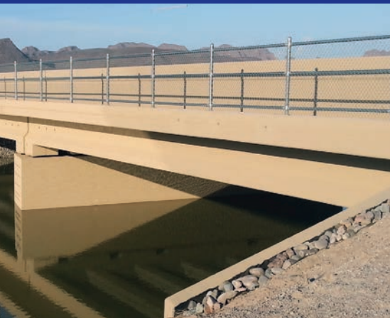
The Sacaton Bridge was replaced using the Innovative Bridge Designs toolkit and was the first "bridge slide" project used by a tribal nation. | Photo courtesy Gila River Indian Community
