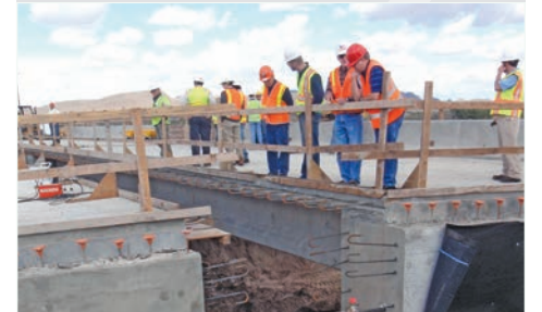
Engineers observe the "side-slide" bridge project at the Gila River Indian Community in Sacaton, AZ during a showcase event for Innovative Bridge Designs for Rapid Renewal . | Photo courtesy Finn Hubbard, Fish & Associates
