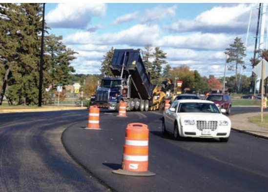
Wisconsin DOT applies a pavement preservation treatment using the Guidelines for the Preservation of High-Traffic-Volume Roadways. | Photo courtesy WisDOT
