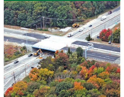
The completed Warren Ave Bridge, Providence, RI | Photo courtesy RIDOT
