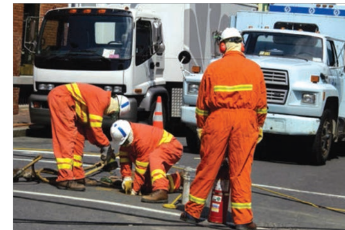
Gas company employees repairing a utility line on a road in Alexandria, VA | Photo courtesy Liz Roll, FEMA
