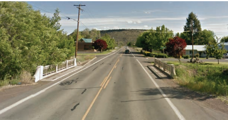
The Ochoco Creek Bridge in Prineville, OR that will be replaced using Managing Risk in Rapid Renewal Projects . | Photo courtesy Lea Ann Hart-Chambers, Oregon DOT
