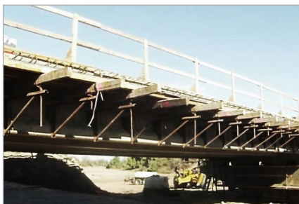
Gila River Slide-In Bridge
