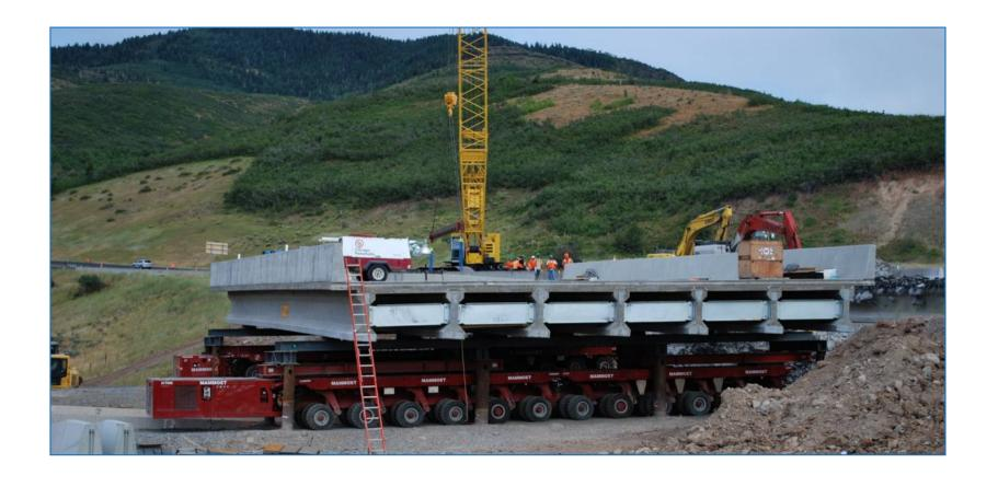
2 Superstructures replaced in 16 hours (including demolition of old bridges)
