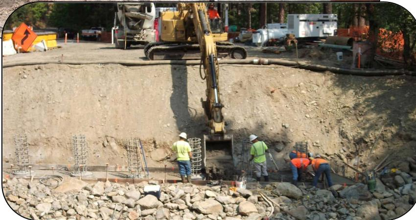
4 sac slurry for abutment bearing pad proved an effective leveling pad.
