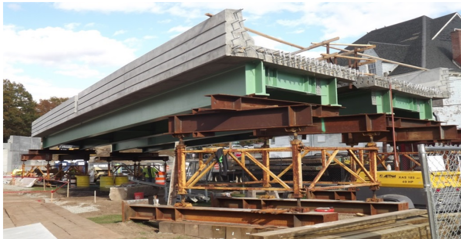
Figure 3. Superstructure ready to be picked up and swung into place on Warren Avenue project, Providence, RI.
