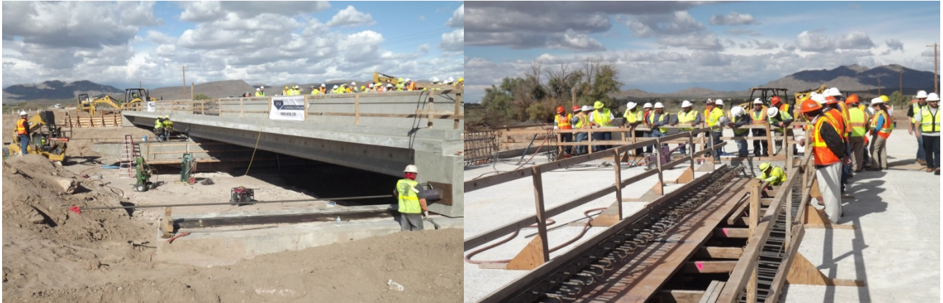
Figure 1. Highly successful CMGC bridge slide, February 2015, at the Gila River Indian Community, Sacaton, AZ.
