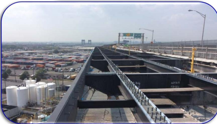
NB section of the Skyway prepared for the installation of the precast deck panels
