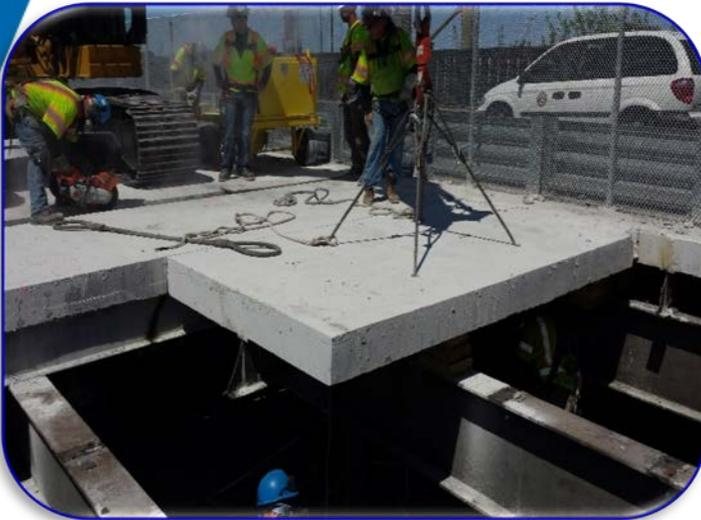
Contractor began removing the existing NB concrete deck in May 2014
