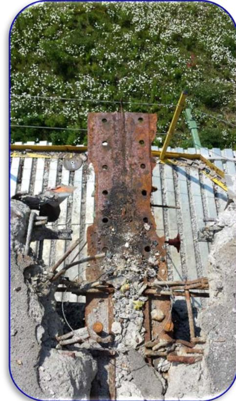
Severe deterioration of top flange of the existing floor beam
