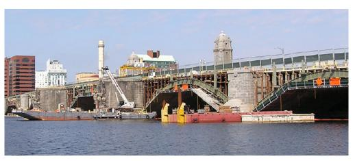
Looking toward Cambridge, ongoing work on the Longfellow Bridge shows the salt and pepper shakers on the upstream side removed to street level.
