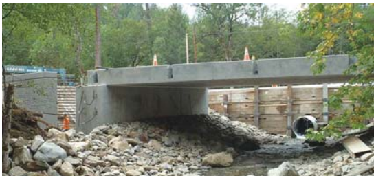
Precast concrete elements are connected by grouted keyways, post-tensioned tie rods, and closure placements.
