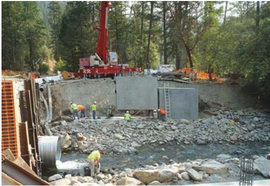
A cement slurry provided an excellent leveling pad for quick and accurate placement of 85-kip abutment segments.
