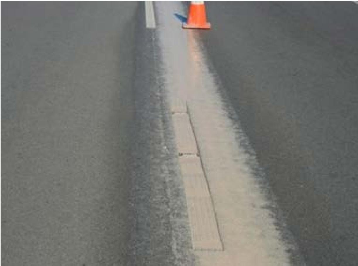
**Figure 4. JointBond Longitudinal Joint Stabilizer within Minutes of Application (Source: KYTC)**
