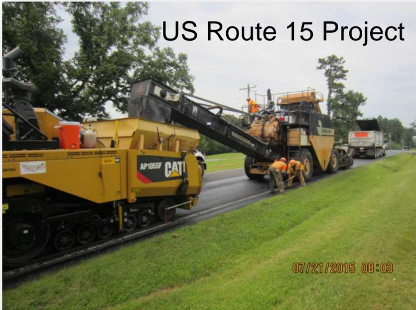
Mixture placed with Caterpillar paver. MTV used on the US Route 15 project.
