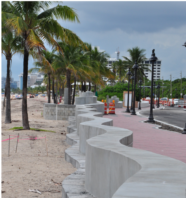
The Florida Department of Transportation (FDOT) used an accelerated schedule to deliver reconstructed beach improvements after Hurricane Sandy devastated the area.
