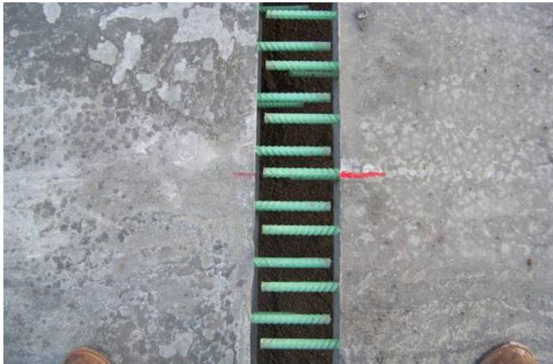
6-inch joint using straight bars
