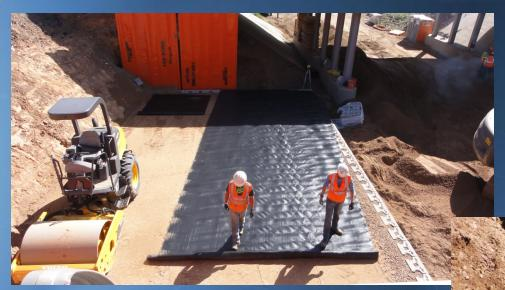
Roll out geosynthetic with strong direction perpendicular to abutment face.
