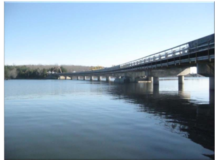
VDOT Route 208 Bridge Deck
