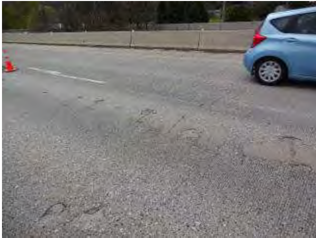
BR08746N: Spalling and Patch Repair
