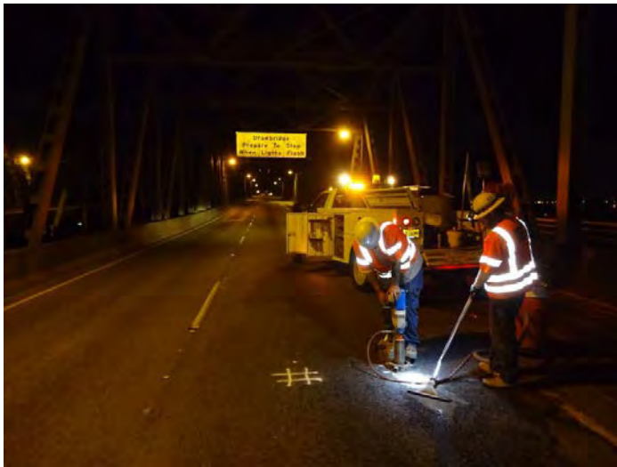
Core Cutting on the Interstate Bridge
