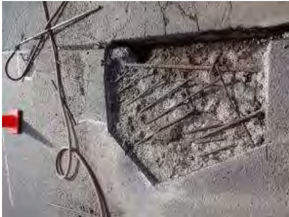
BR09259 Repair Area at Deck-Impact Panel Joint
