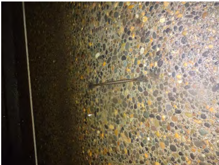
BR08306: Single Exposed Rebar
