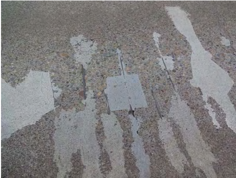
BR08492 Exposed Rebar on Deck
