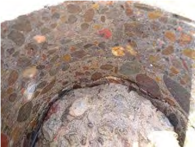
BR09259A: Core Hole Showing Relatively Shallow Portion of Overlay With Corrosion Induced Fracture at Top Mat Plane
