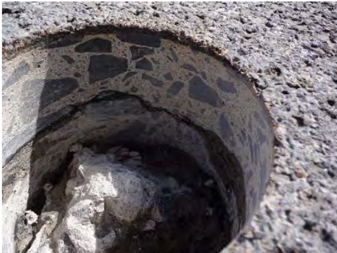
BR08347A: Corrosion Induced Delamination Fracture within Core
