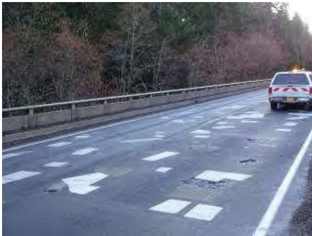
BR2071A: Damage on Deck of Span 1
