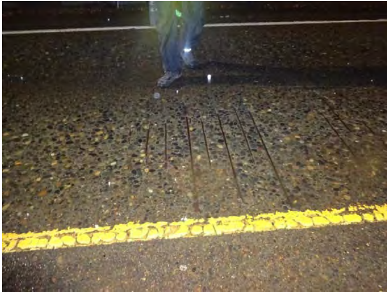
BR08306: Typical Exposed Rebar Pattern
