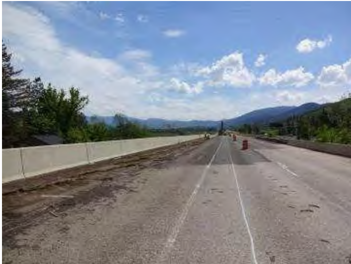
BR08746N: Overview of Right Travel Lane with Spalled/Patched Areas
