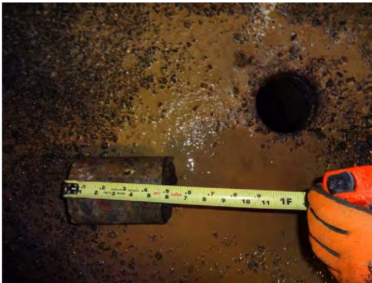
Core Sample Demonstrating 5.5” Deck With Compromised ACWS
