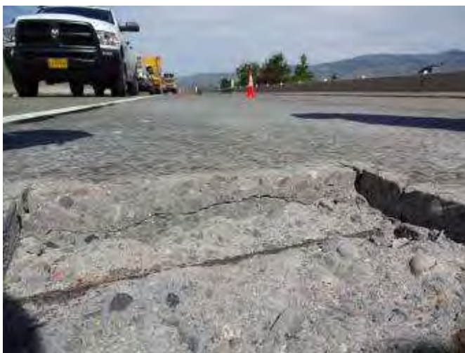
BR08746S: Repair Area Showing Surface Cracking, Corrosion, and Fracture Plane at Rebar Depth
