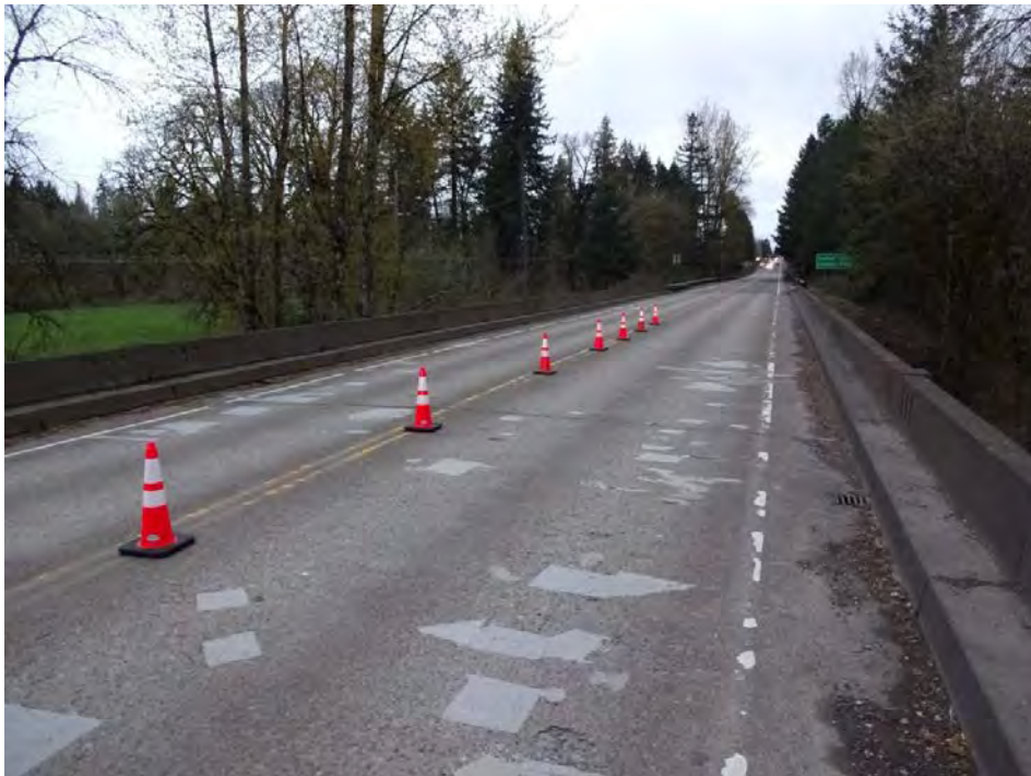
BR08492 Damage on Deck
