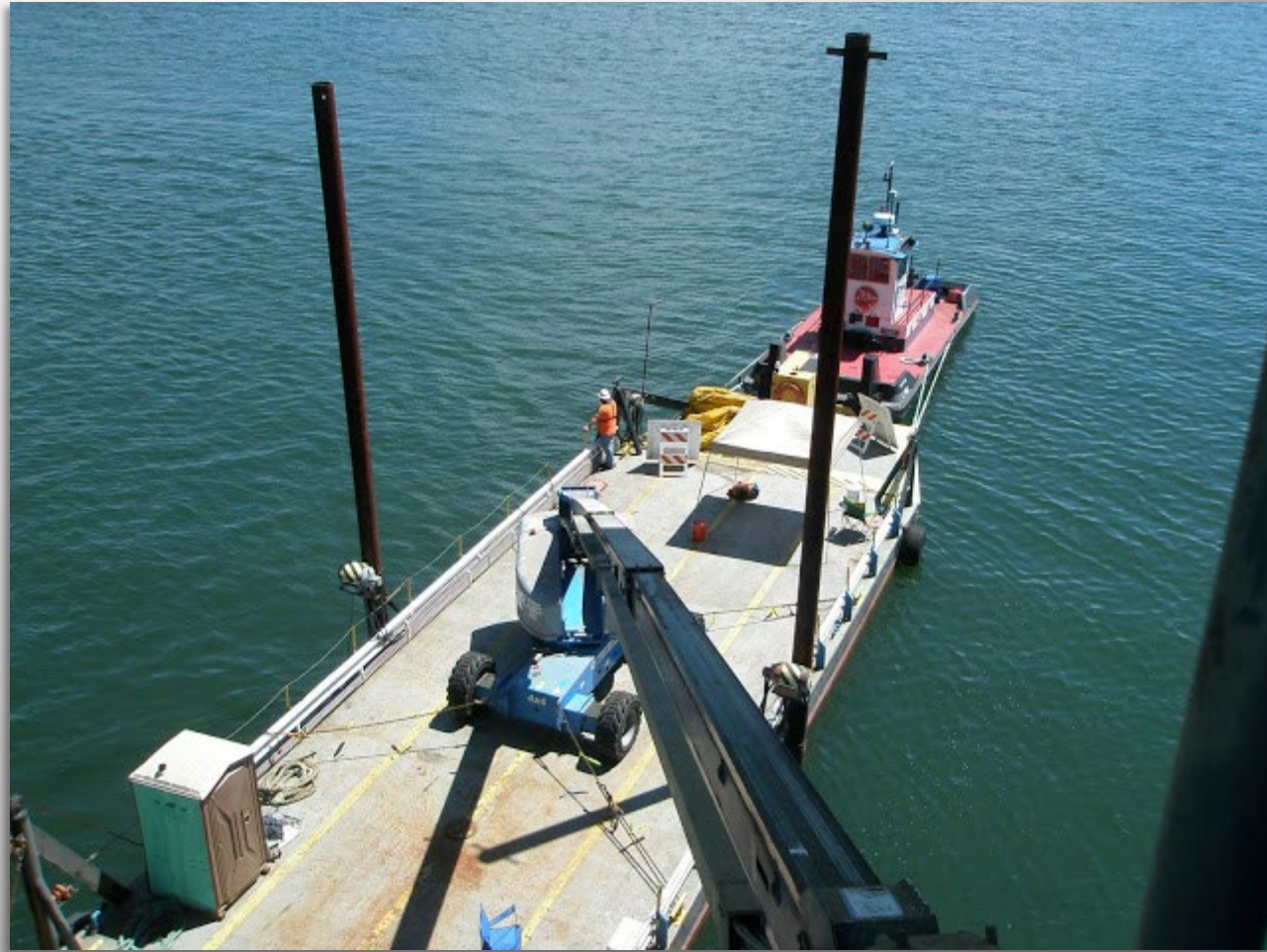
Image 3: FC inspection of NB Interstate Bridge
