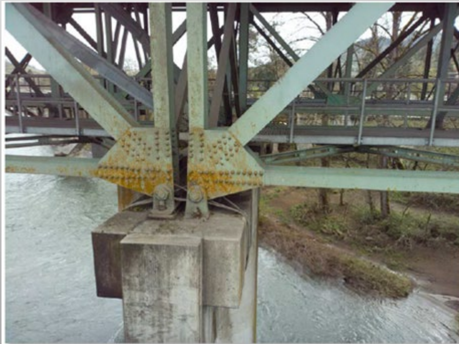
Southern bent pin connection. Taken from senseFly albris main HD camera. Focal length: 8 mm, 35mm equivalent: 25 mm. (Full image)
