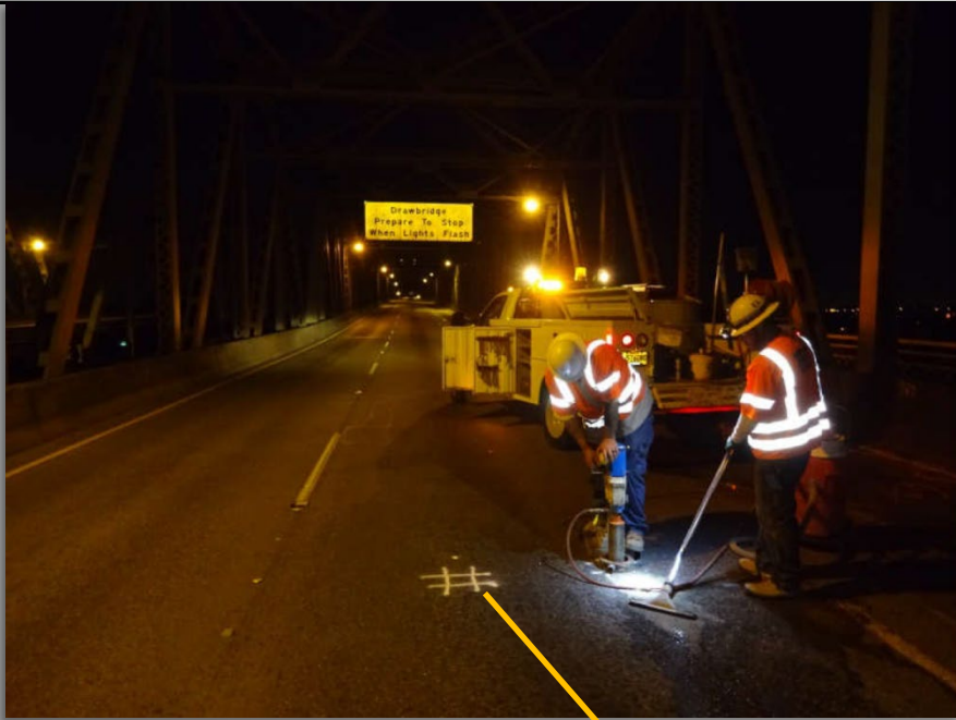
Image 4: Coring the NB Interstate Bridge
