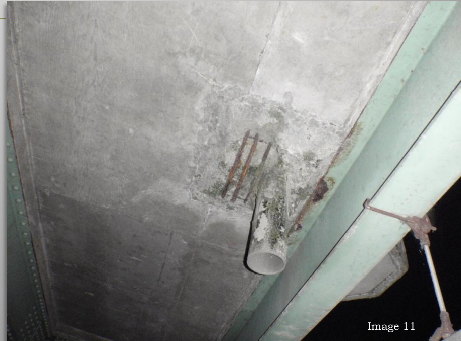
Figure 27 Exposed rebar 1' x 2' 1' x 2' Exposed rebar 1' x 1' 1' x 1' spall 1' x 1' No delaminations detected
