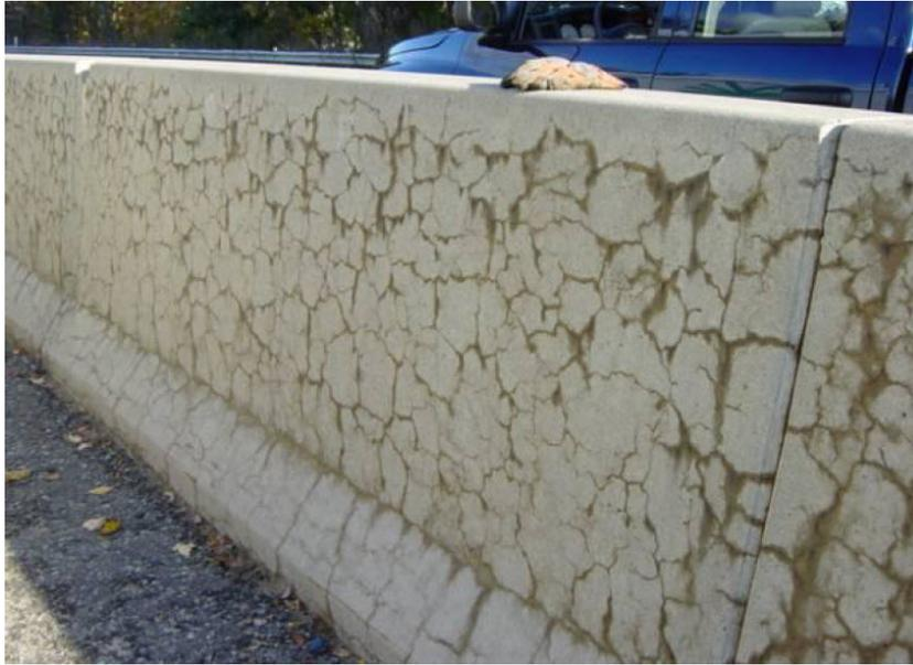
**Figure 8: Concrete barrier attacked by AAR (FHWA, 2010).**
