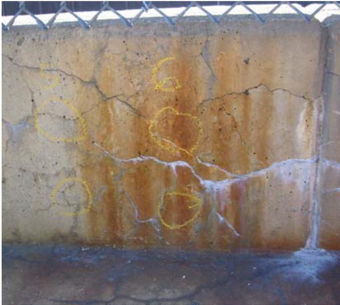
**Figure 7: Delayed ettringite formation in concrete wall (*Characterization of Delayed Ettringite Formation in Maryland Bridges*, dissertation by Micah Shalom, 2007).**
