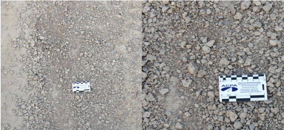
**Figure 10: Scaling of concrete pavement exposed to freeze-thaw and de-icing salts (FHWA, 2015).**
