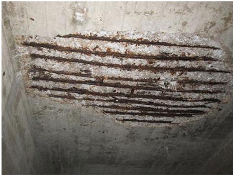
**Figure 14: Corrosion of the underside of an existing bridge deck (FHWA, 2014).**
