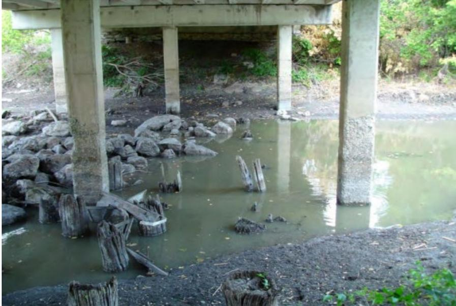
**Figure 6: Sulfate attack of concrete piers in contact with sulfate bearing water (FHWA, 2010).**
