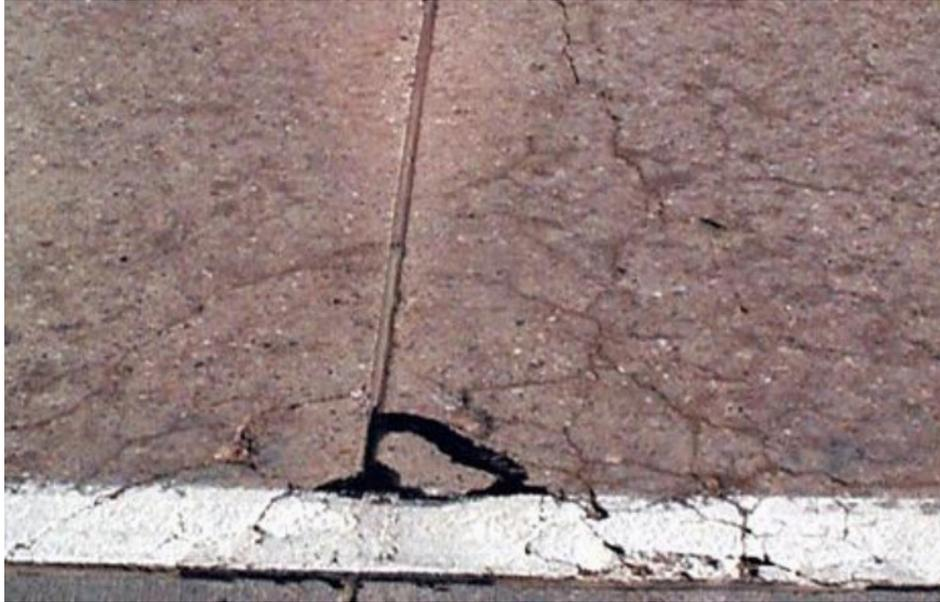
**Figure 9: Internal cracking of concrete pavement exposed to freeze-thaw (FHWA, 2015).**
