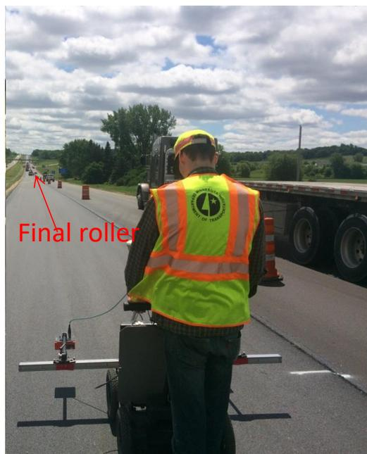
**Figure 6: Rolling Density Meter Surveying Behind Final Roller**
