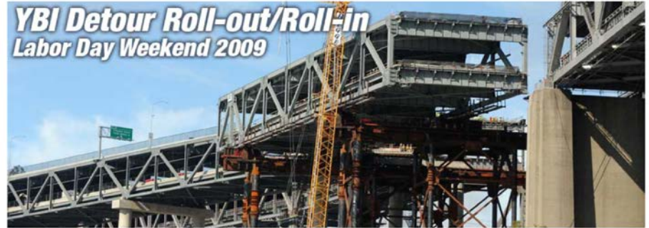
SFOBB Yerba Buena Island Viaduct superstructure roll-in
