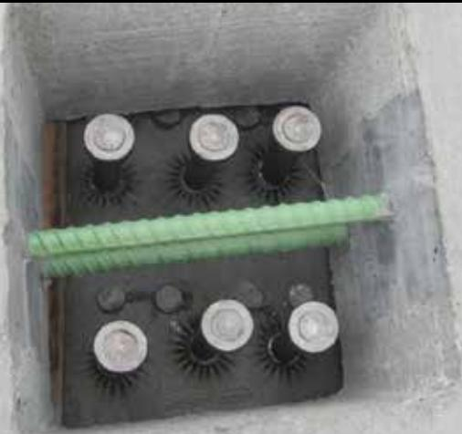
P/T Duct Connection at Panel Joint
