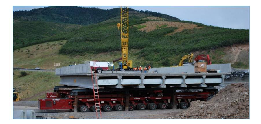
2 Superstructures replaced in 16 hours (including demolition of old bridges)
