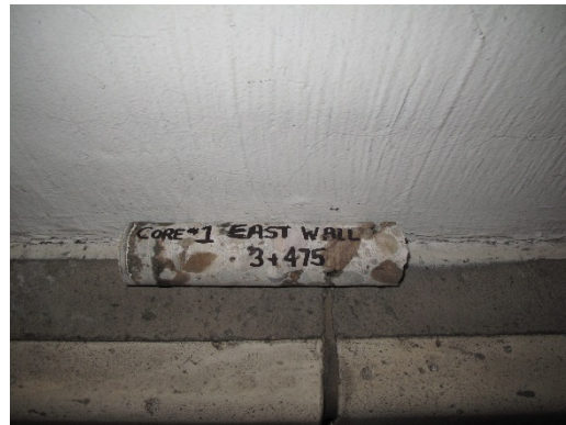
Photo 23: Extracted Core, Station 3+475
