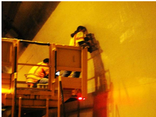
Photo 15: PSPA Testing from Lift Vehicle
