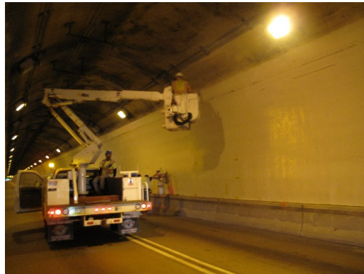
Photo 18: Hammer Sounding Inspection
