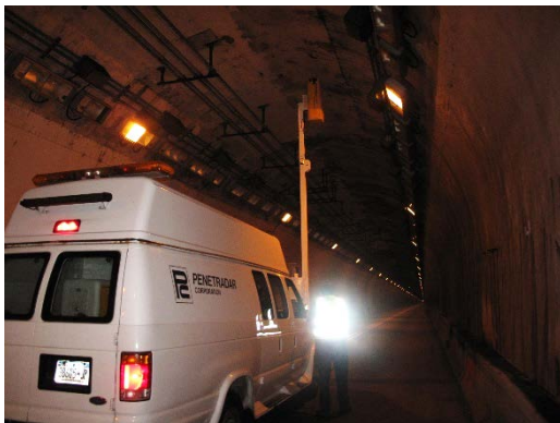
Photo 7: Penetradar GPR Ceiling Scan
