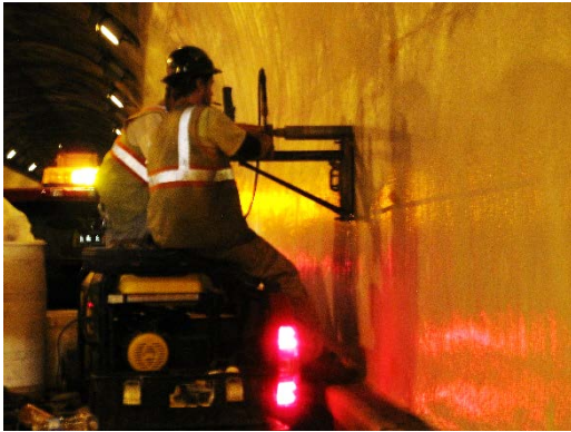
Photo 20: Concrete Coring, Station 3+321
