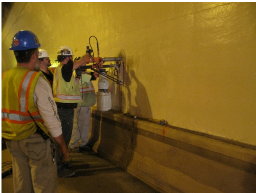
Photo 22: Concrete Coring, Station 3+475
