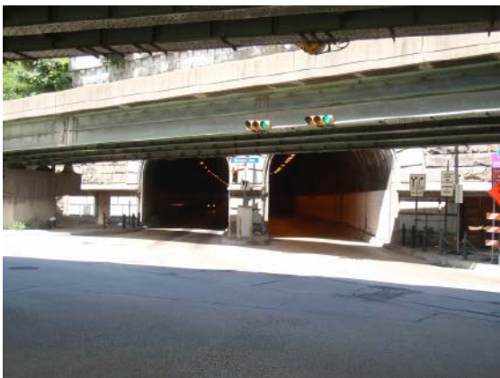
Photo 3: Armstrong Tunnel South Entrance
