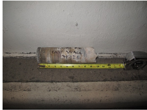
Photo 21: Extracted Core, Station 3+321
