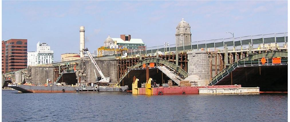
*Looking toward Cambridge, ongoing work on the Longfellow Bridge shows the salt and pepper shakers on the upstream side removed to street level.*
