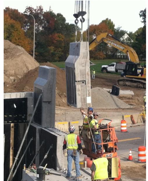
*South Abutment, Placing Wingwall Precast Concrete Element (PCE), 10/30/2014*
