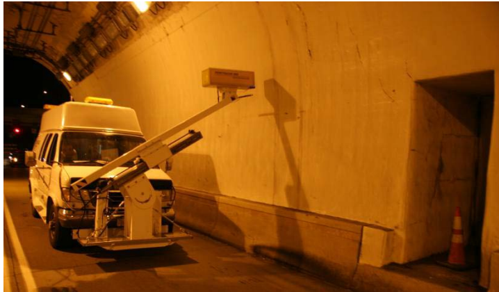
Penetrator GPR of PennDOT Tunnel
