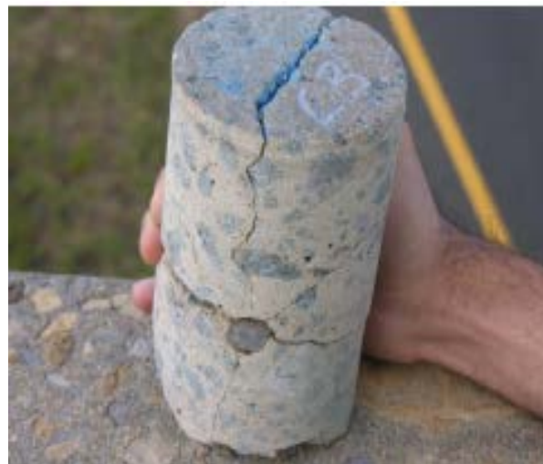
C3 - delamination at 3.5 inches
