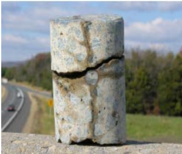
C5 - delamination at 2.5 inches
