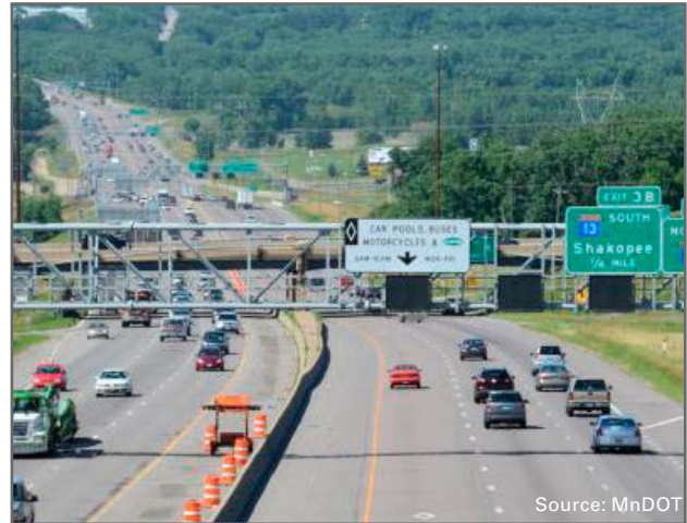
MnDOT used Reliability Data and Analysis Tools to address congestion and travel-time reliability.
