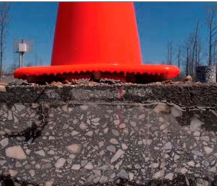
GPR can help detect delamination in hot-mix asphalt.
