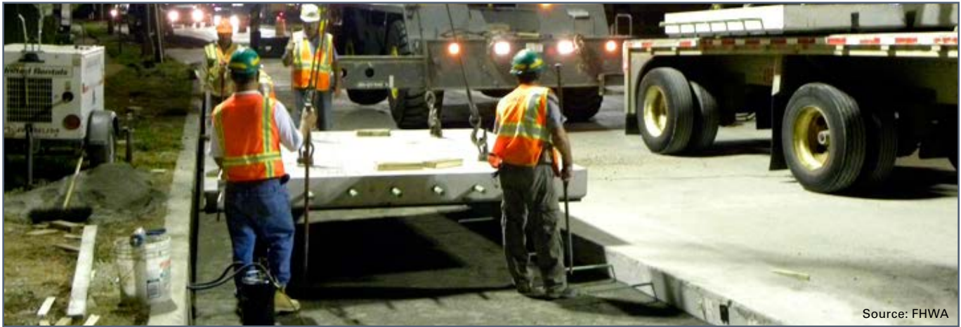
PCP installation at an intersection along Rockaway Boulevard in New York.
