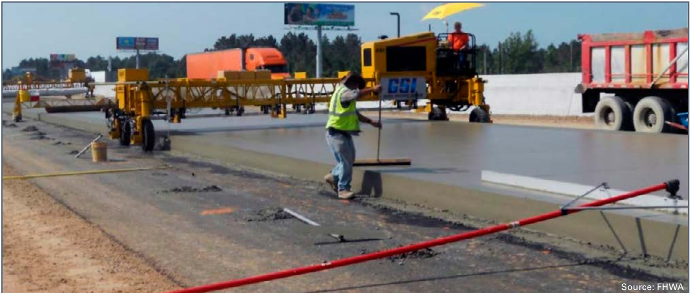
Real-time smoothness measurements (self-propelled work bridge). Source: FHWA
