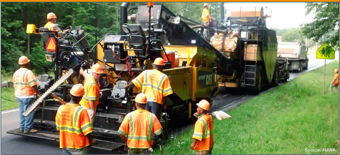
Using NDT infrared technology on asphalt pavements in Virginia.
