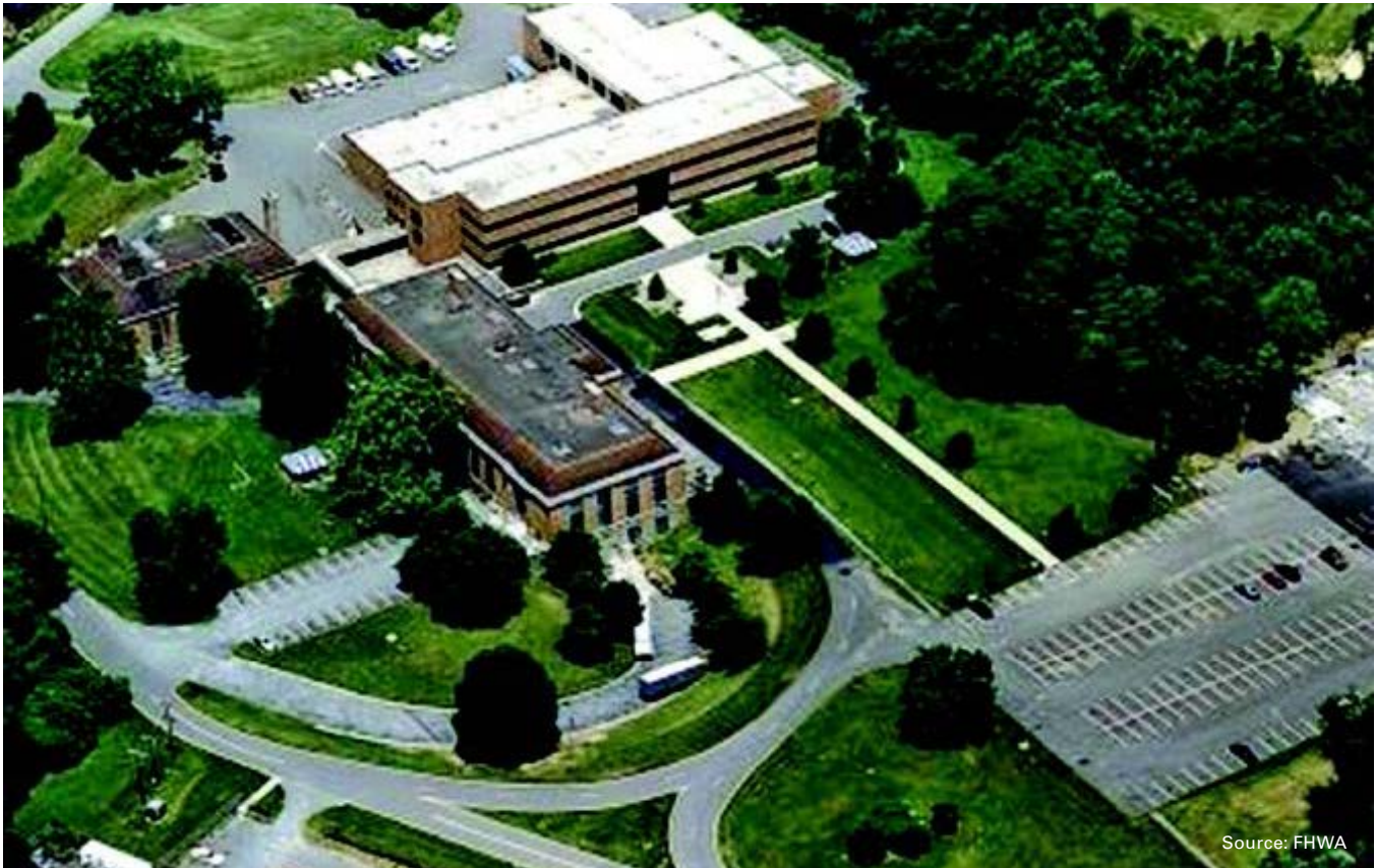
The Safety Training and Analysis Center is located at the Turner-Fairbank Highway Research Center.
