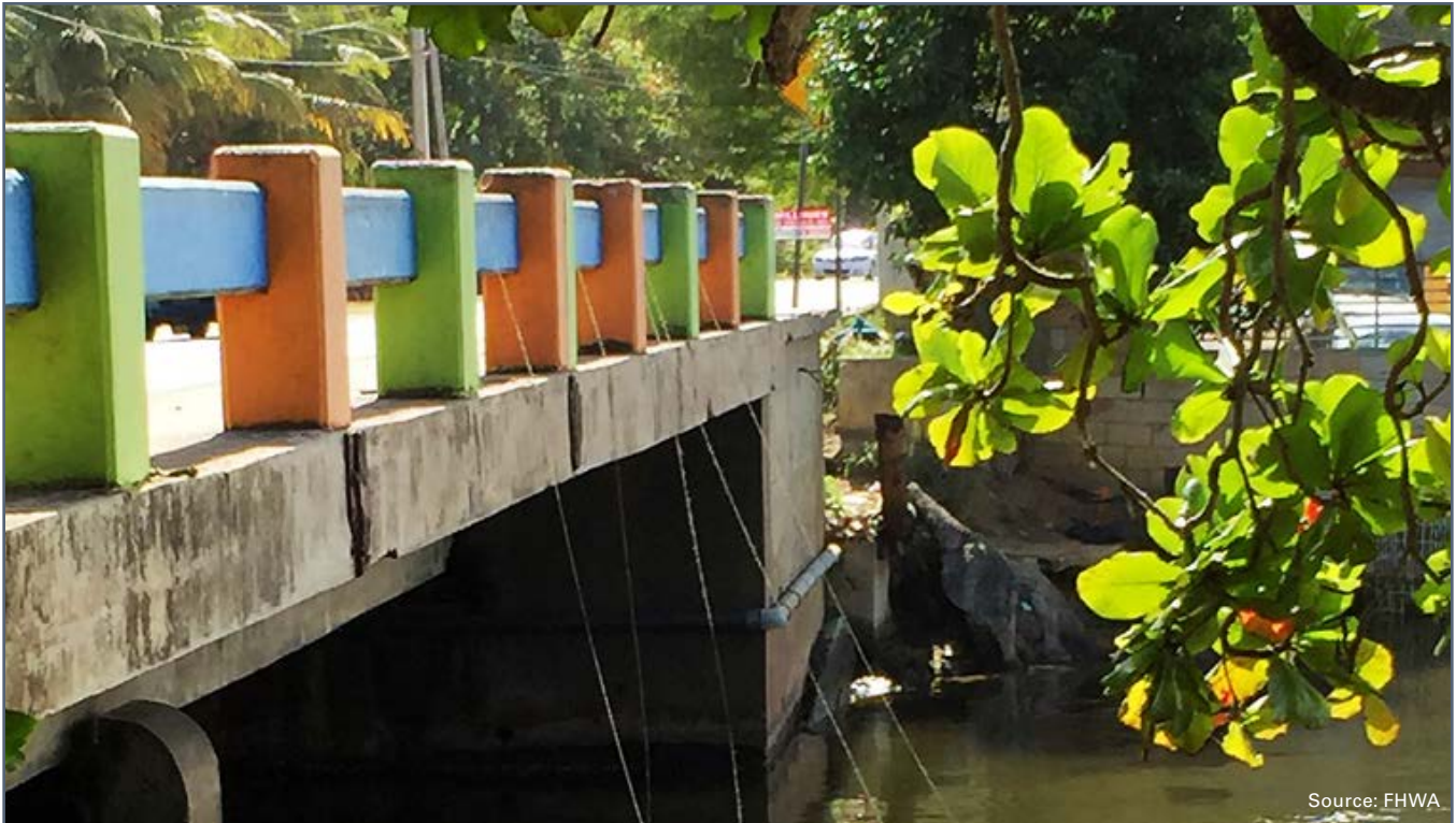
Bridge 702 on Puerto Rico Route 681 before Arecibo, Puerto Rico.
