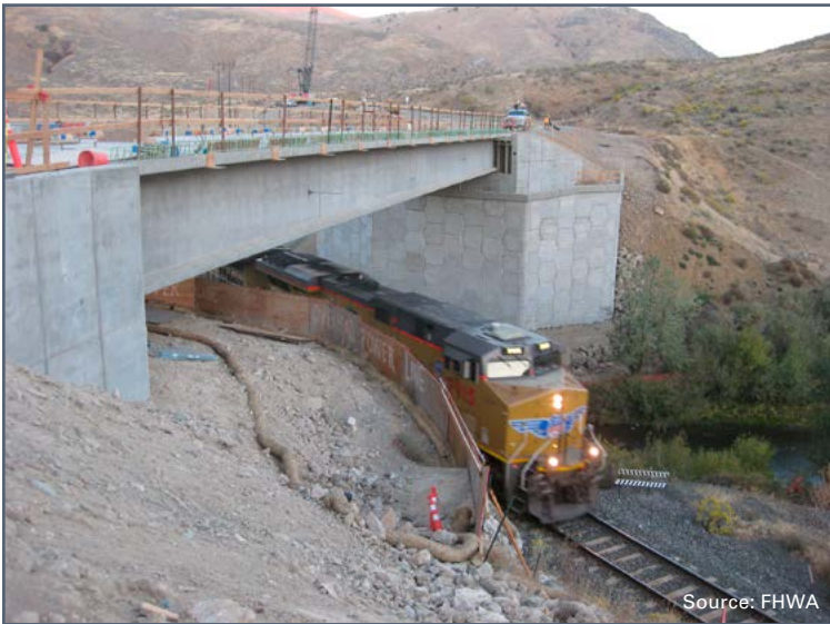
Bridge removal project north of Ontario, Oregon on US 30.
