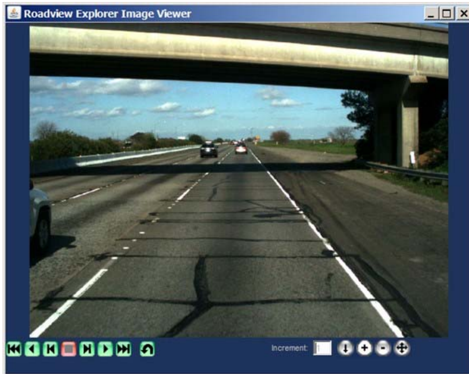
Figure 7-2 A photo of a JPCP truck lane taken at PM 32.55 EB of the Solano project.
