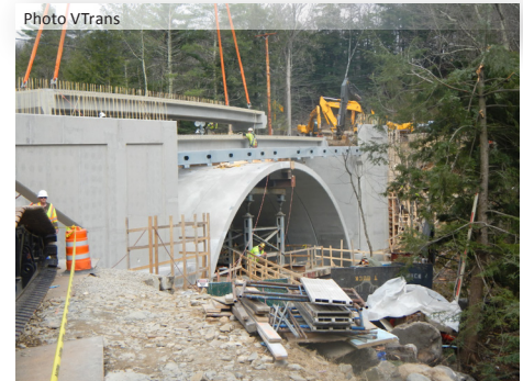
Collaboration strategies led to significantly shortened road closures during bridge construction.
