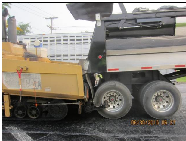
Figure 12. End-Dump Truck Delivering Mixture to Caterpillar Paver on the IL 116 Project
