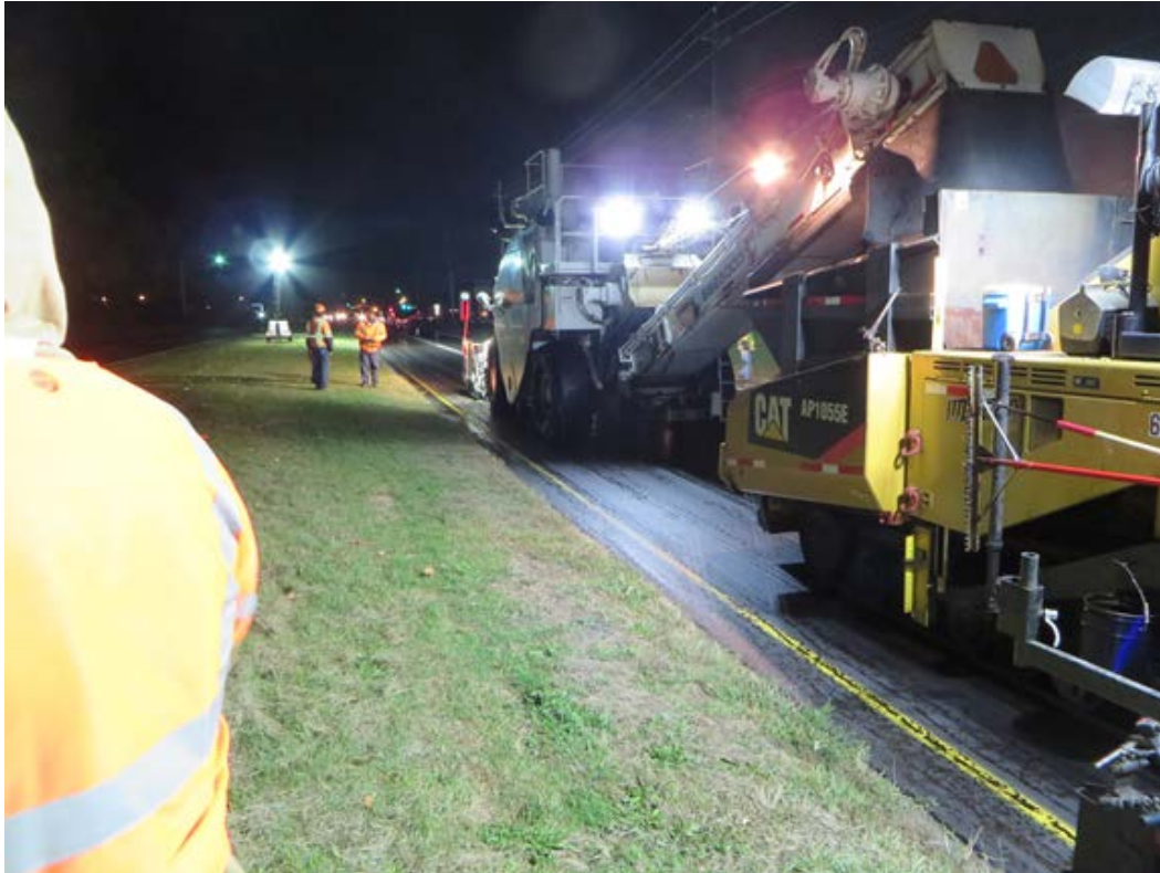
Figure 20. Paving Operation Used along the New Jersey US-130 Project Location.
