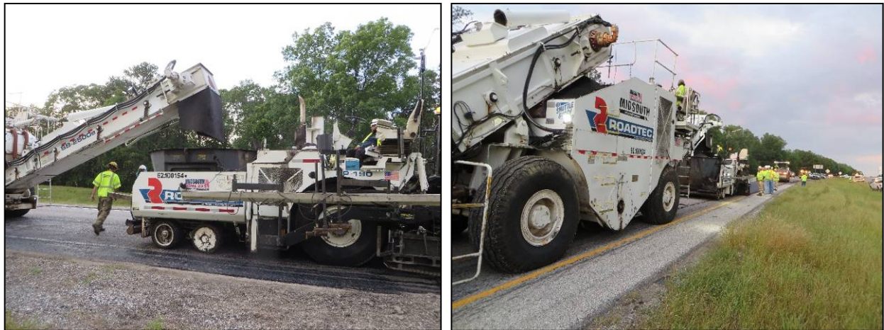
Figure 4. Roadtec Paver and Roadtec Material Transfer Vehicle Used to Place the Mixture.
