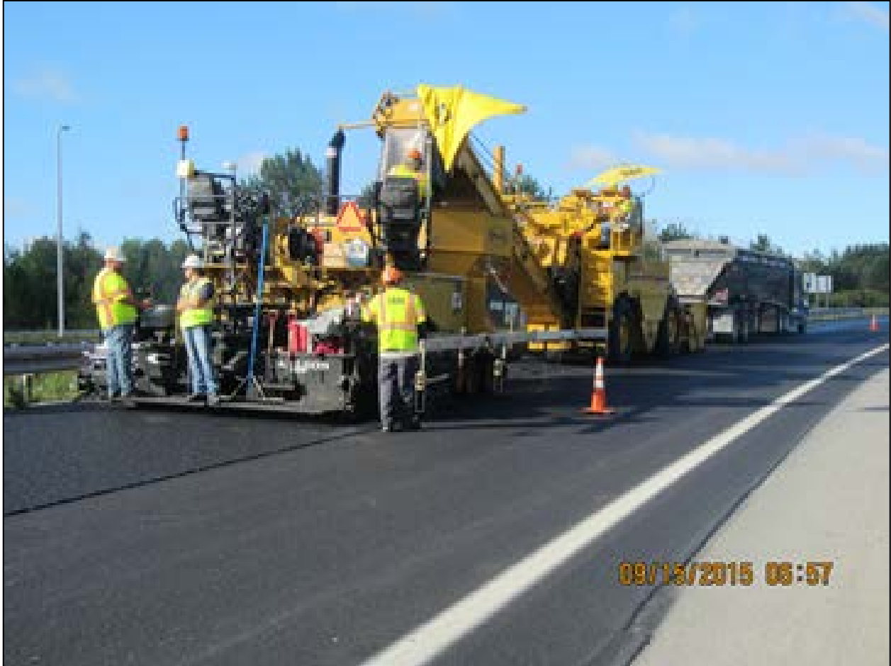
Figure 16. Paving Operation Used along the Maine I-95 Project
