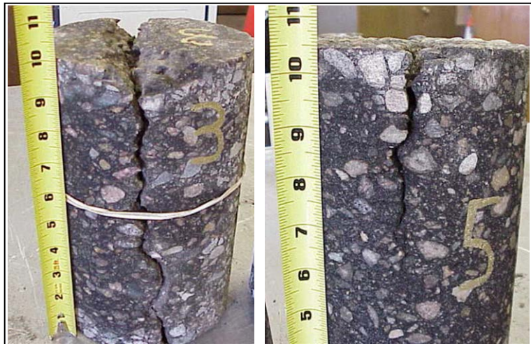
Figure 1. Longitudinal Aggregate Segregation and Top-Down Cracking.
