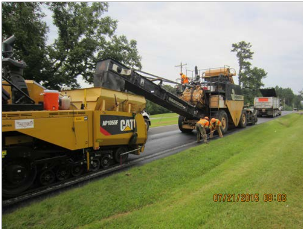
Figure 24. Delivery-Paving Operation Used along the Virginia US-15 Project.
