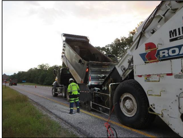
Figure 3. End-Dump Trucks Delivering Mixture to the Alabama Paving Site.
