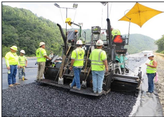
Figure 27. Placement of Drainage Base on the Geosynthetic Fabric along State Route 10
