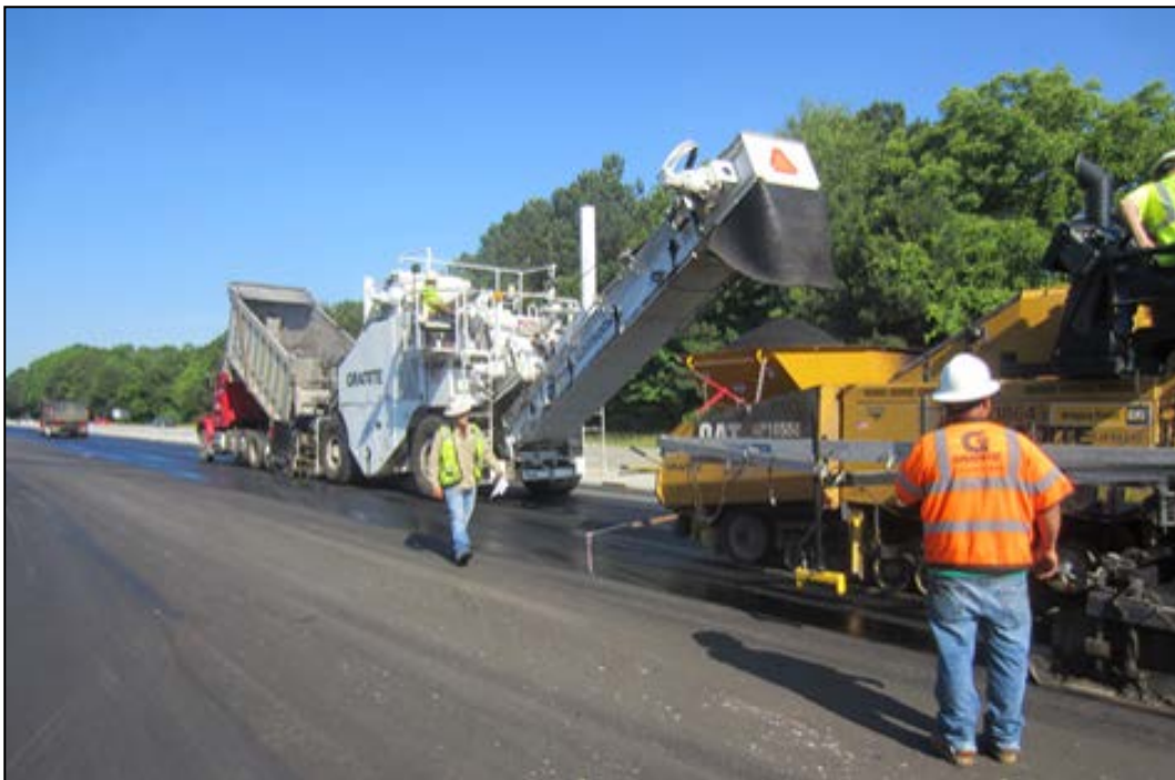
Figure 22. Paving Operation Used along the North Carolina I-40 Project.
