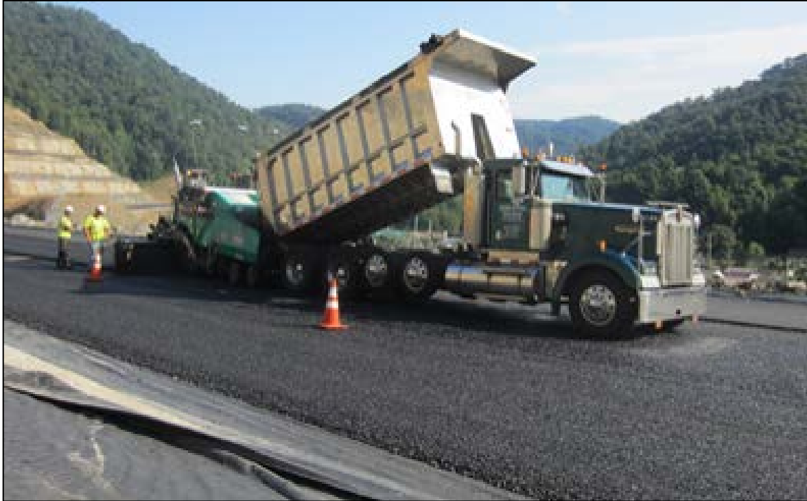
Figure 26. Mixture Delivery-Paving Operation used along the State Route 10 Project
