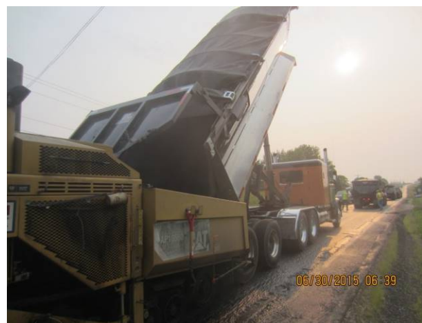
Figure 12. End-Dump Truck Delivering Mixture to Caterpillar Paver on the IL 116 Project
