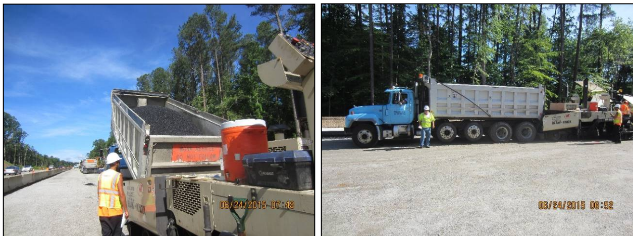
Figure 9. End-Dump Trucks Delivering Mixture to the EFL Paving Site
