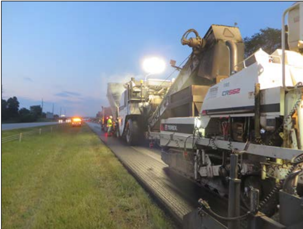
Figure 18. Paving Operation Used along the Missouri I-29 Project.
