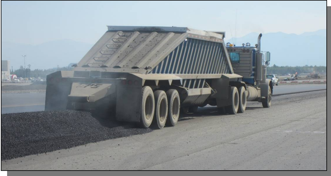
Figure 7. Bottom-Dump Truck Delivered Mix to Alaska Paving Site.
