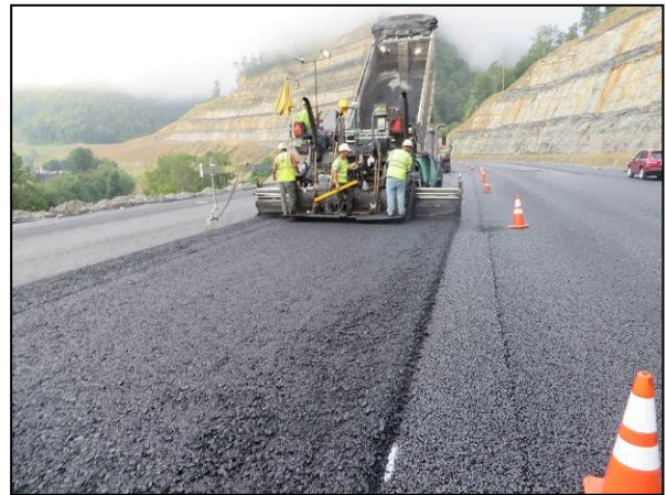
Figure 27. Placement of Drainage Base on the Geosynthetic Fabric along State Route 10
