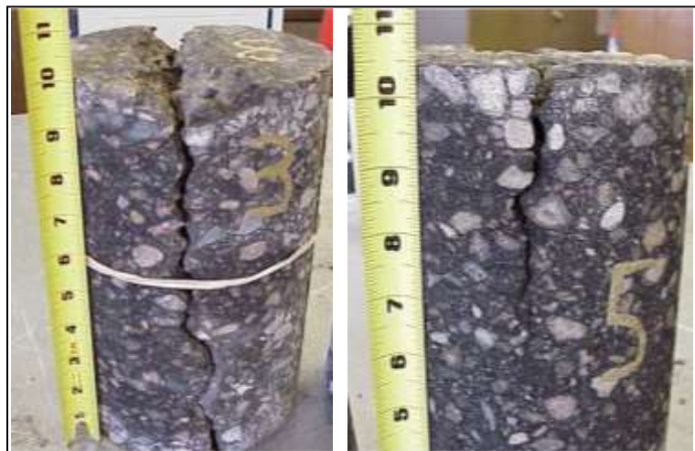
Figure 1. Longitudinal Aggregate Segregation and Top-Down Cracking
