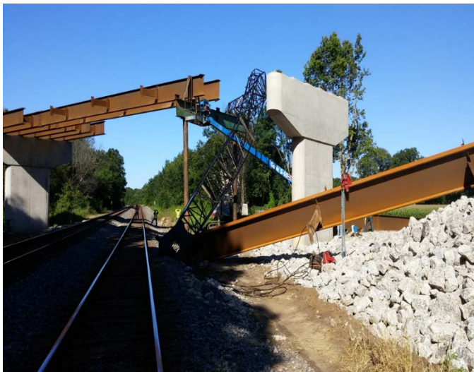
Example of work requiring a flagger
