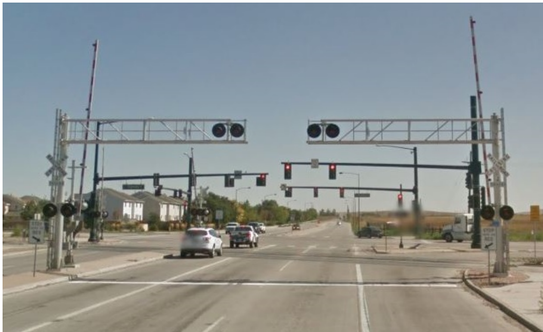
Figure 3-12: 96 th Avenue at Highway 2 Presignal, Henderson
