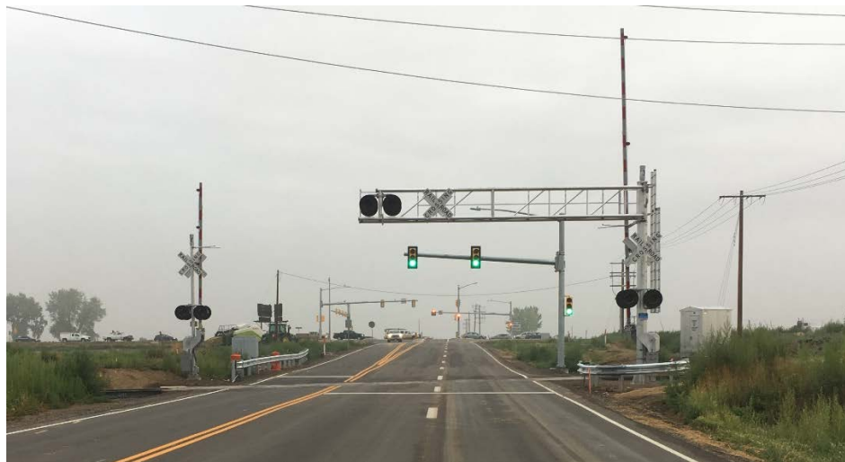
Figure 3-14: Weld County Road 13 at Great Western Railway, Weld County
