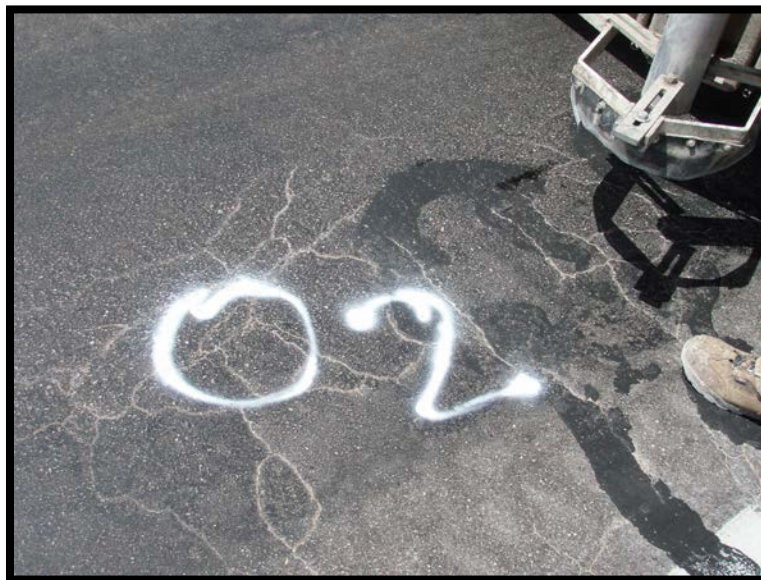
Figure 3.7: Marked Location on I-10 (WB) for Core #2 (MP 365)
