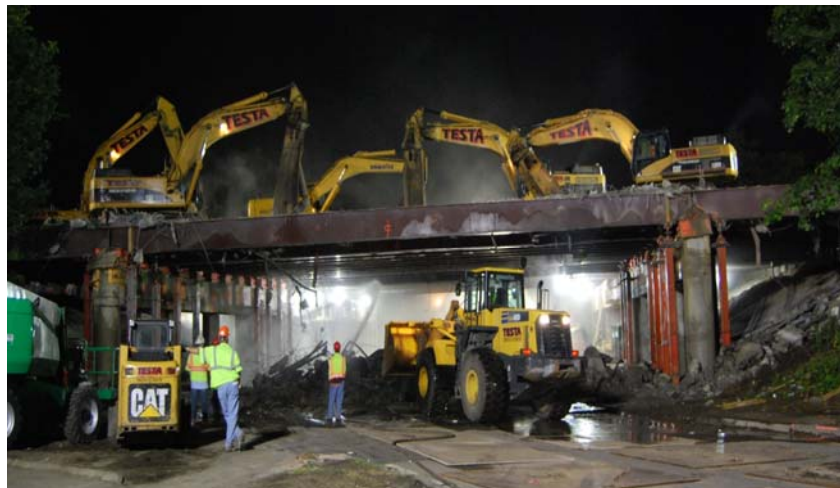
Fast 14 Project – Friday night, 10 PM, Demolition Starts
