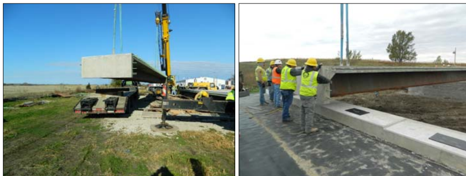
Nebraska Department of Roads place girder/deck units
