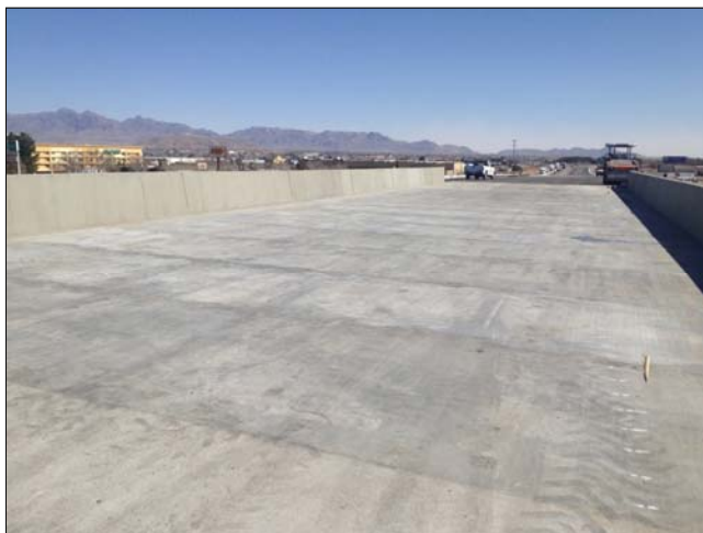
Panels after Placement
