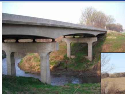
Old Keg Creek Bridge
