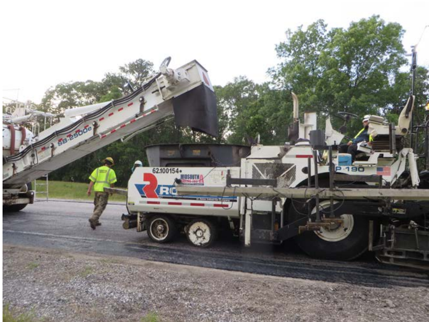
Mixtures placed with Roadtec Rubber Tired Paver
