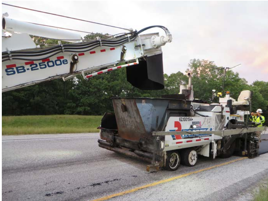
Roadway without tack coating applied
