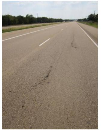
Thermal streaks can be very damaging, depending on the level of density achieved in localized areas.
